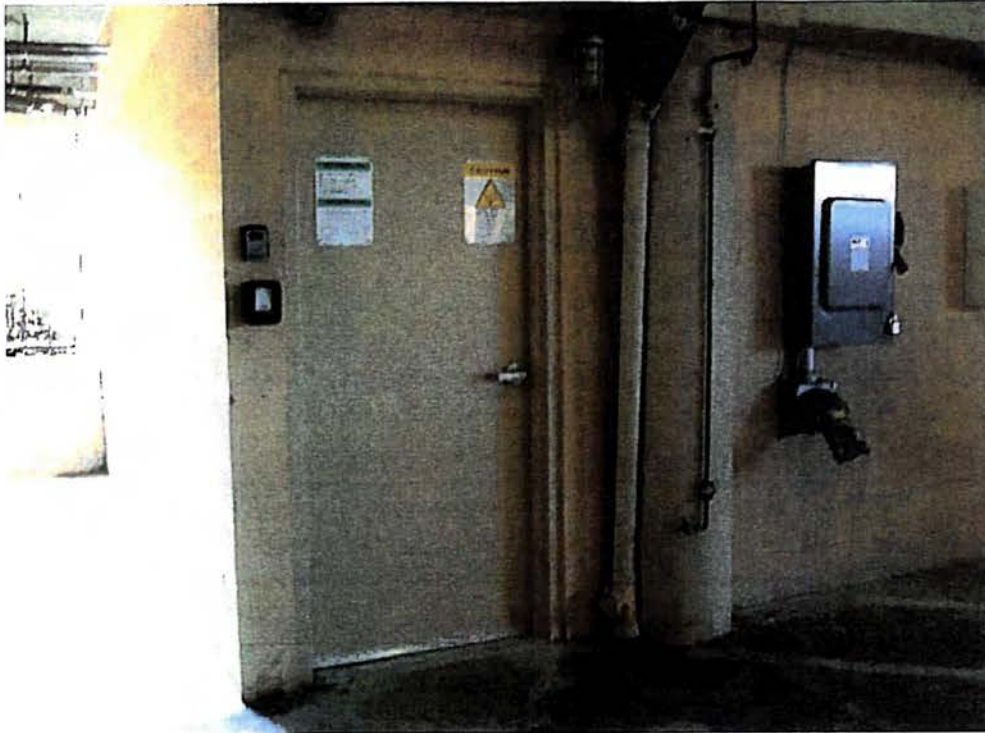
Existing Equipment Room
