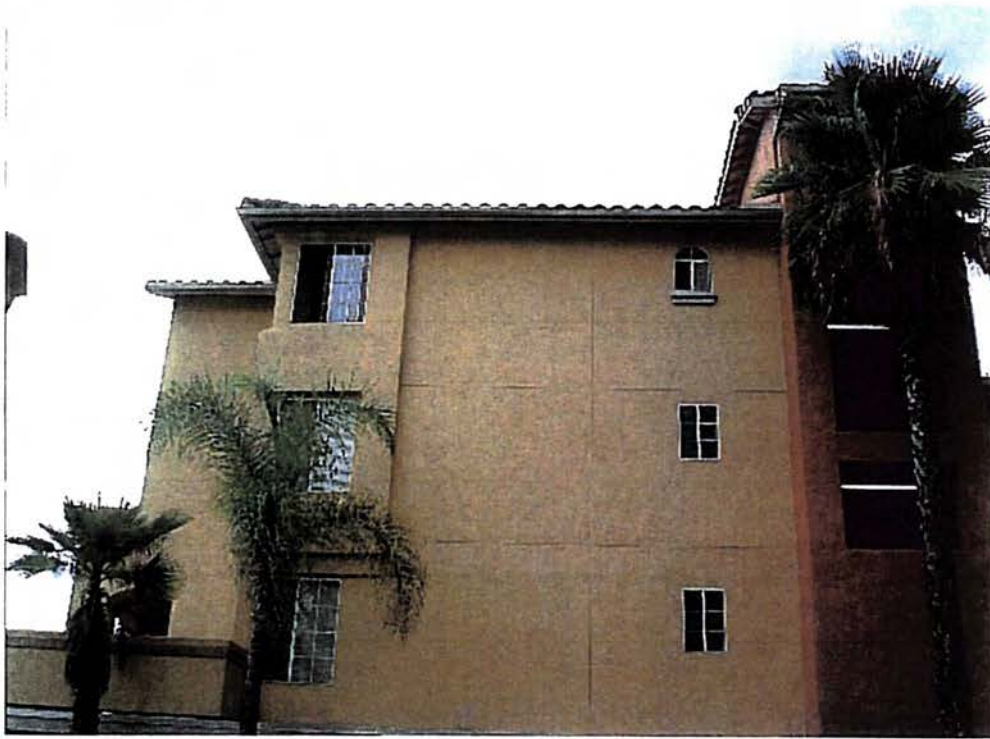
Looking at East Elevation
