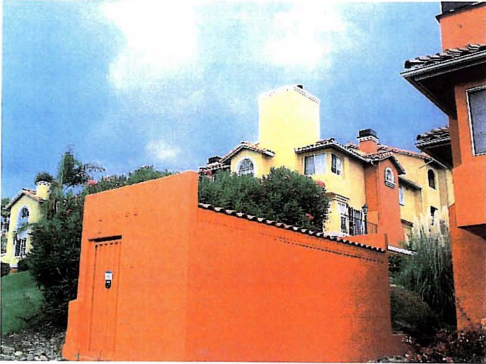
Looking Northeast at site
