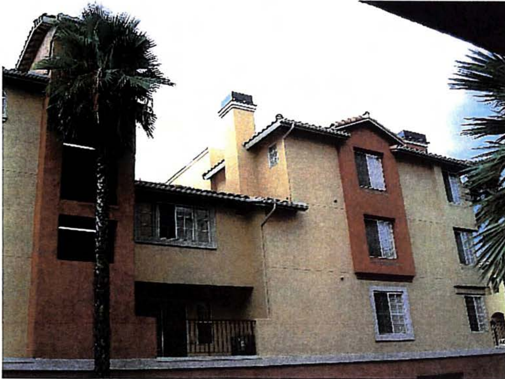
Looking at East elevation
