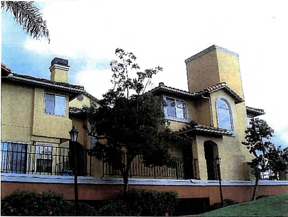
Looking at West elevation
