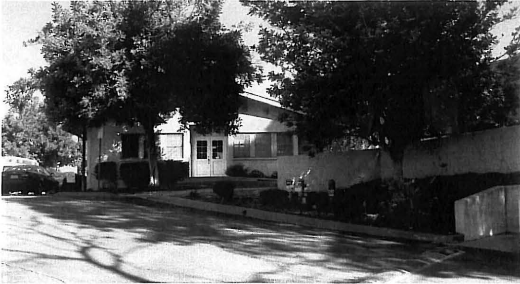
Southwestern corner of existing structure
