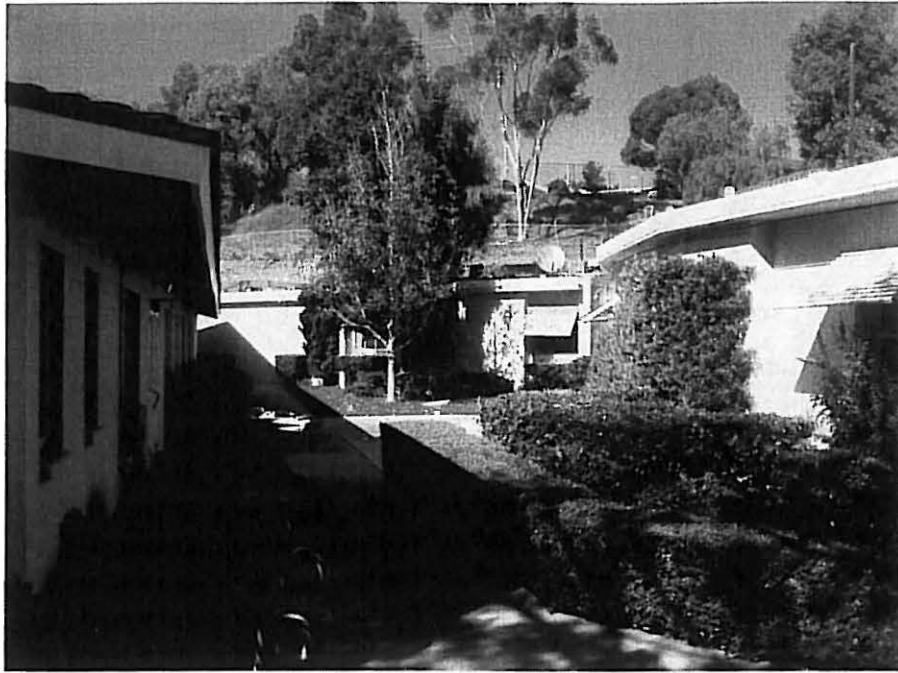
Internal courtyard area of existing structure
