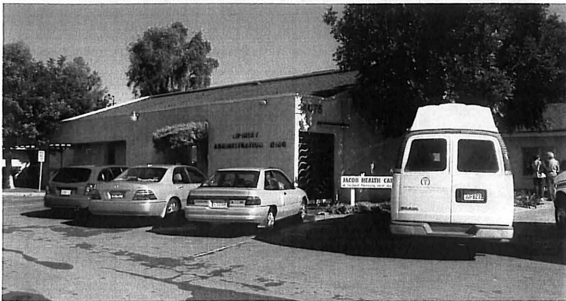
Northwest elevation of existing structure
