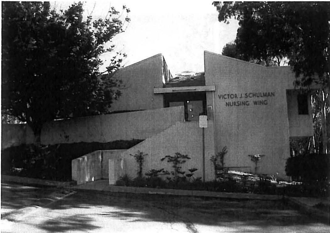
View of west elevation of existing structure when entering from driveway on 54 th Street
