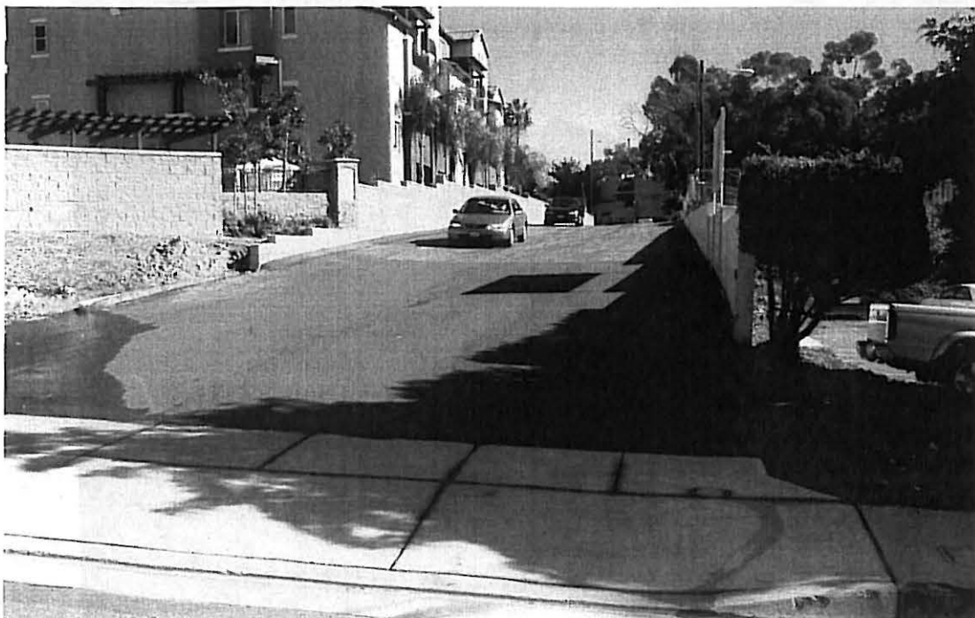
Project Driveway on 54 th Street, Looking East
