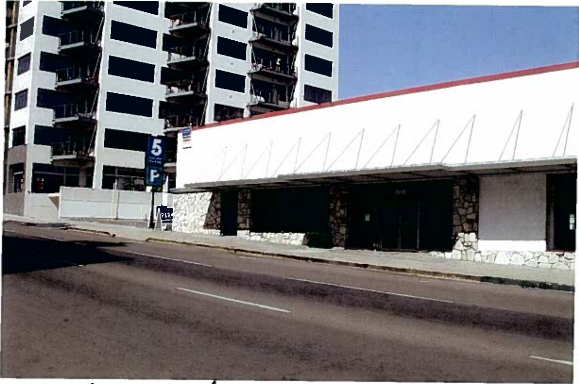
Project to north
