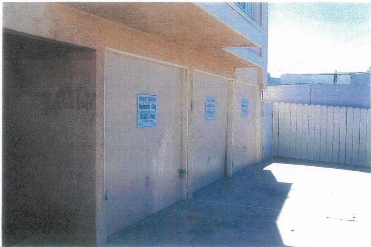
4. REAR OF BUILDING LOOKING SOUTH.
