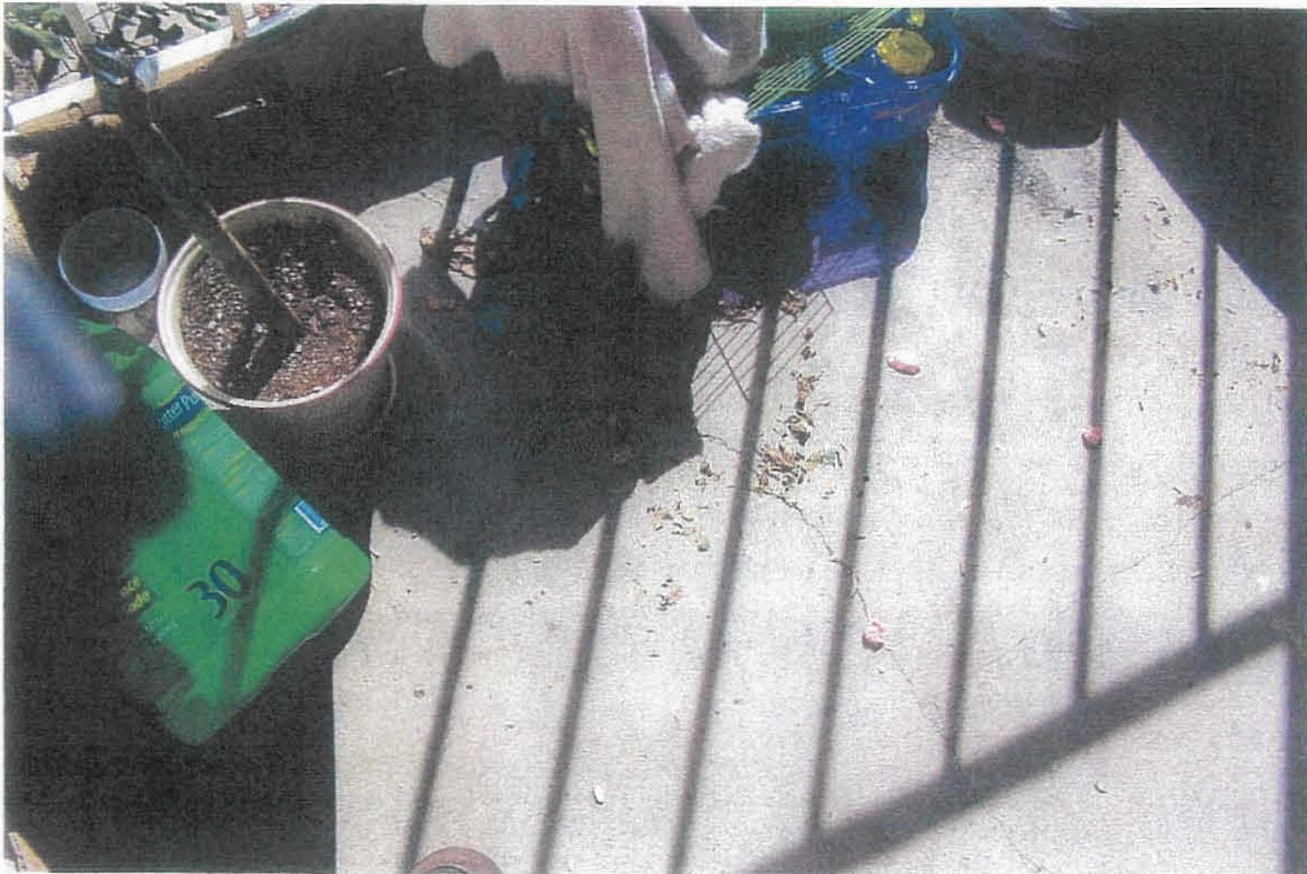
12. TYPICAL SECOND FLOOR BALCONY, NOTE CRACKING.
