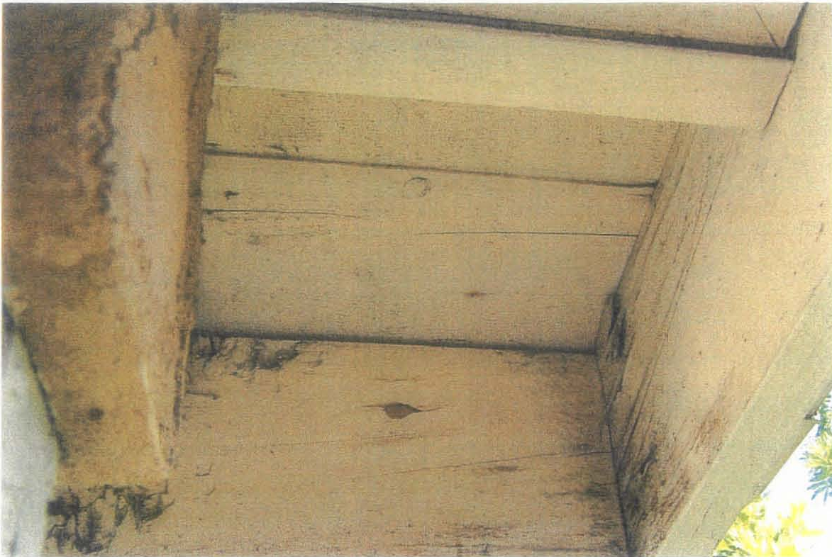
16. MINOR DETERIORATION OF FASCIA BOARDS.
