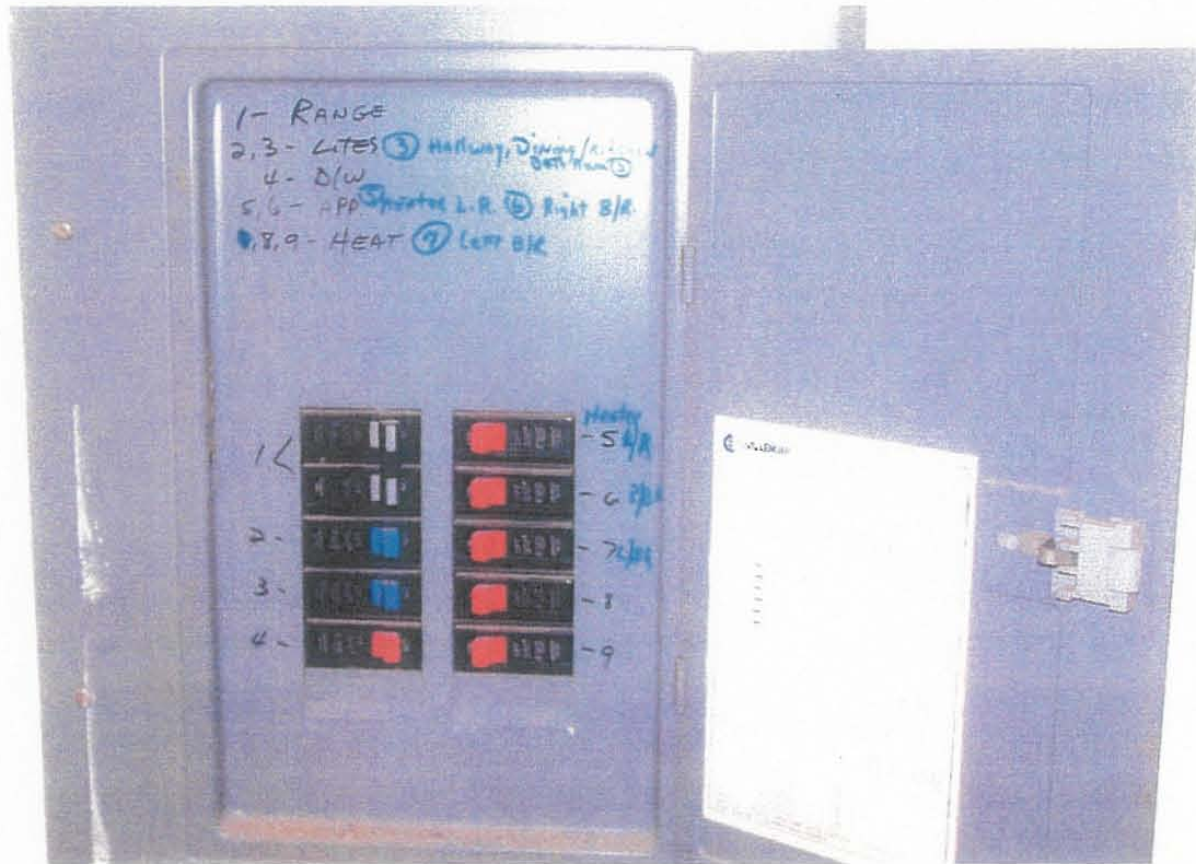
7. CIRCUIT PANEL IN BEDROOM.
