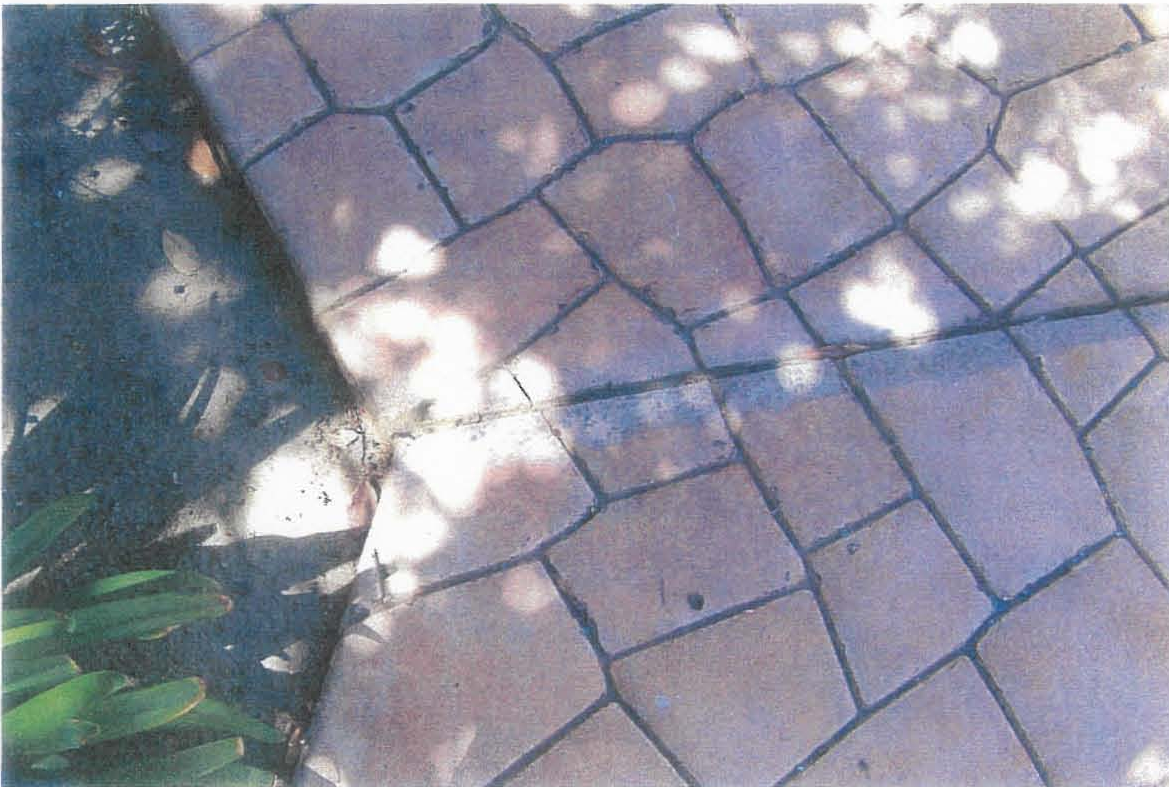
26. TYPICAL SIDEWALK SLAB CRACKS & TRIPPING HAZARDS.
