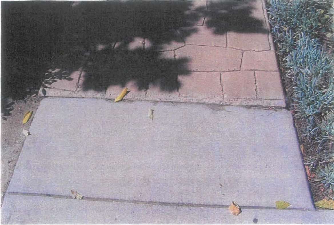
25. TYPICAL SIDEWALK SLAB CRACKS & TRIPPING HAZARDS.
