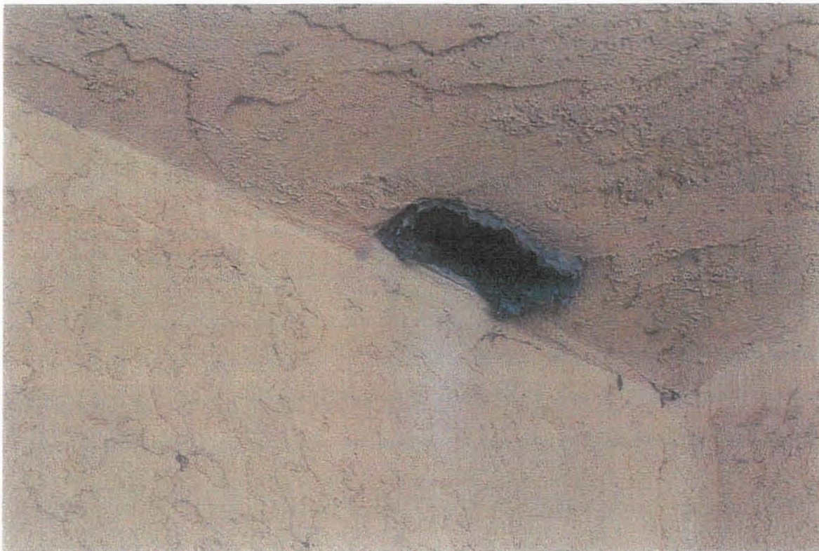
18. LAUNDRY ROOM DRYER VENT MISSING SCREEN.
