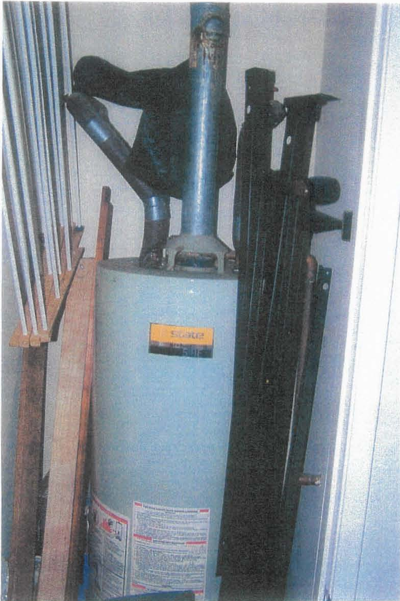
9. TYPICAL, UNSTRAPPED 30 GALLON WATER HEATER.
