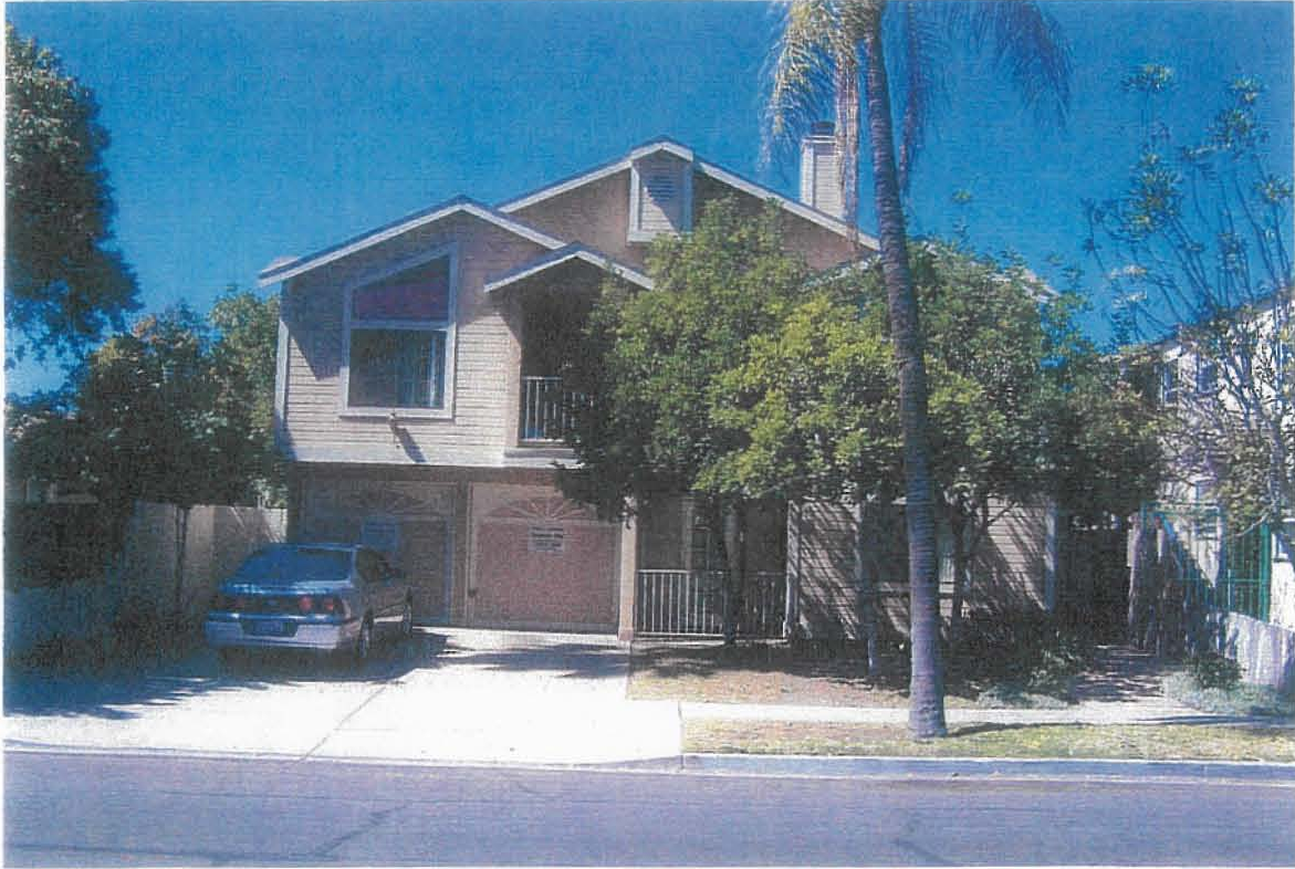
1. FRONT VIEW LOOKING WEST.
