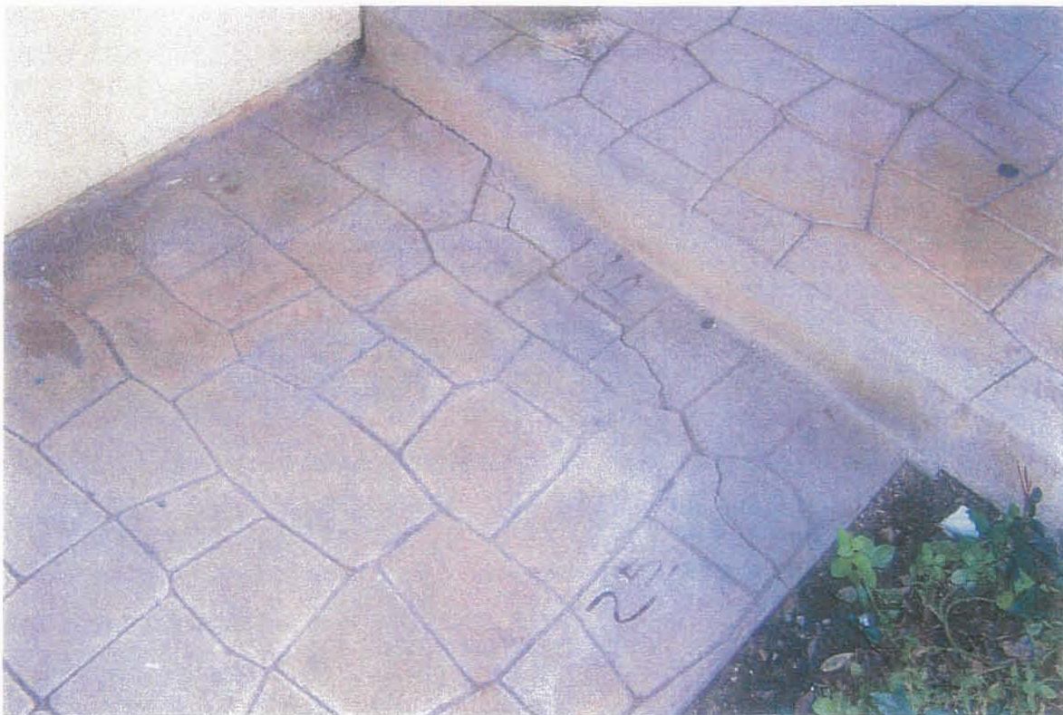
24. TYPICAL SIDEWALK SLAB CRACKS OUTSIDE OF UNITS 1 AND 2.
