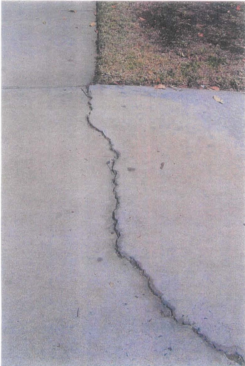
19. DRIVEWAY APPROACH SLAB CRACK AND HEAVING.
