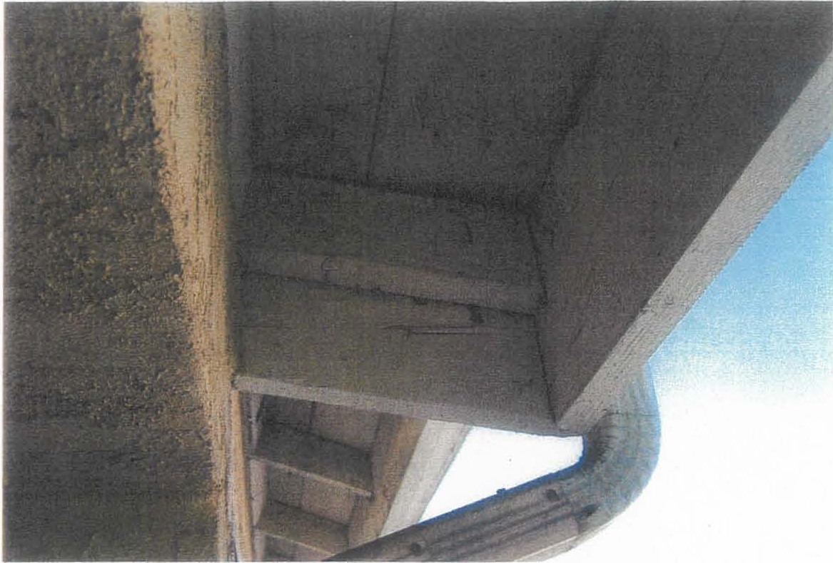
15. MINOR DETERIORATION OF FASCIA BOARDS.
