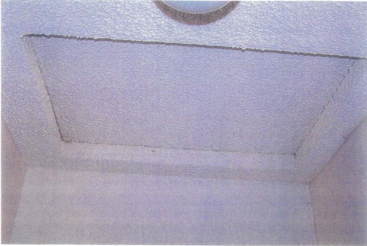
11. ATTIC CRAWL SPACE ACCESS DOOR IN HALLWAY.
