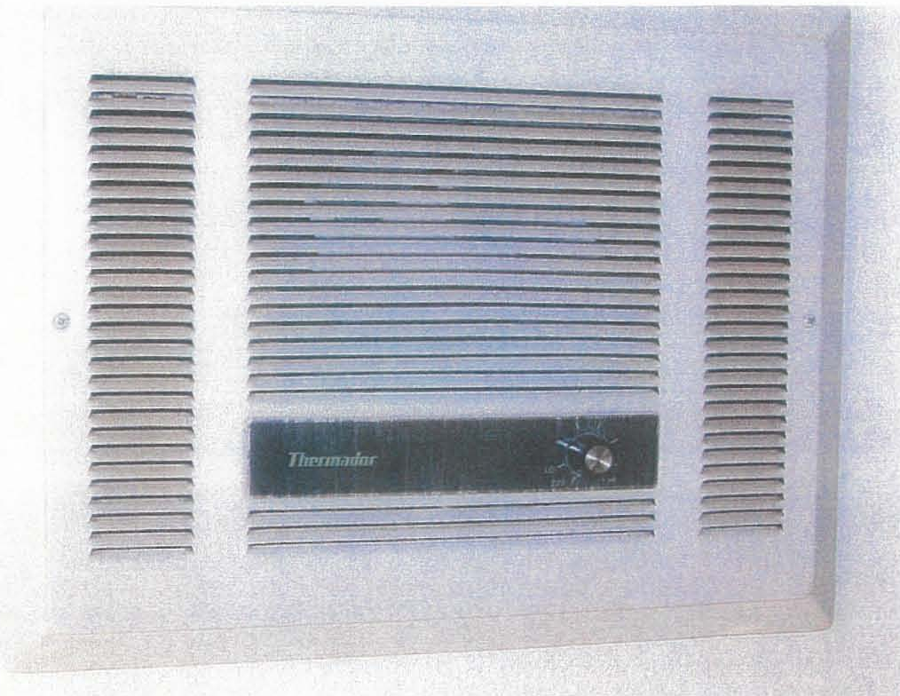
8. ELECTRIC WALL HEATER IN BEDROOMS AND LIVINGROOM.
