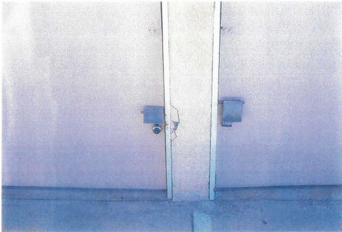
17. TYPICAL STUCCO DAMAGE AROUND GARAGE DOORS.
