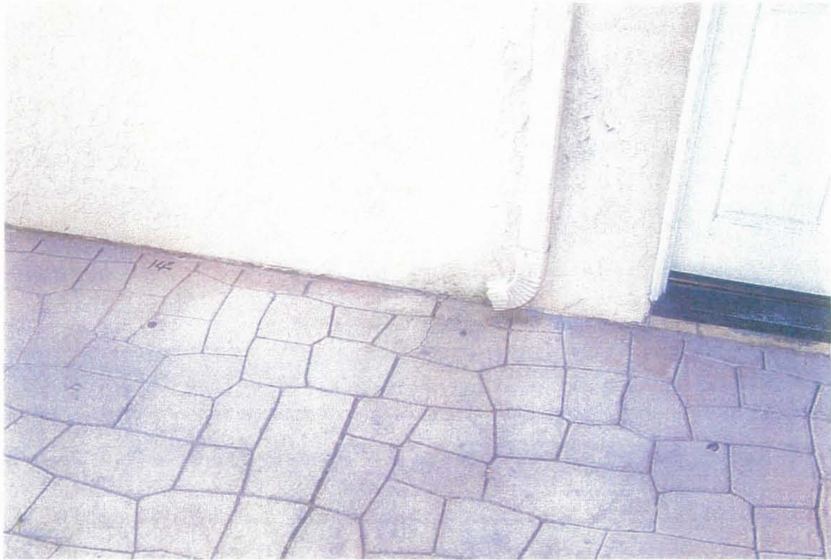
23. TYPICAL SIDEWALK SLAB CRACKS OUTSIDE OF UNITS 1 AND 2.
