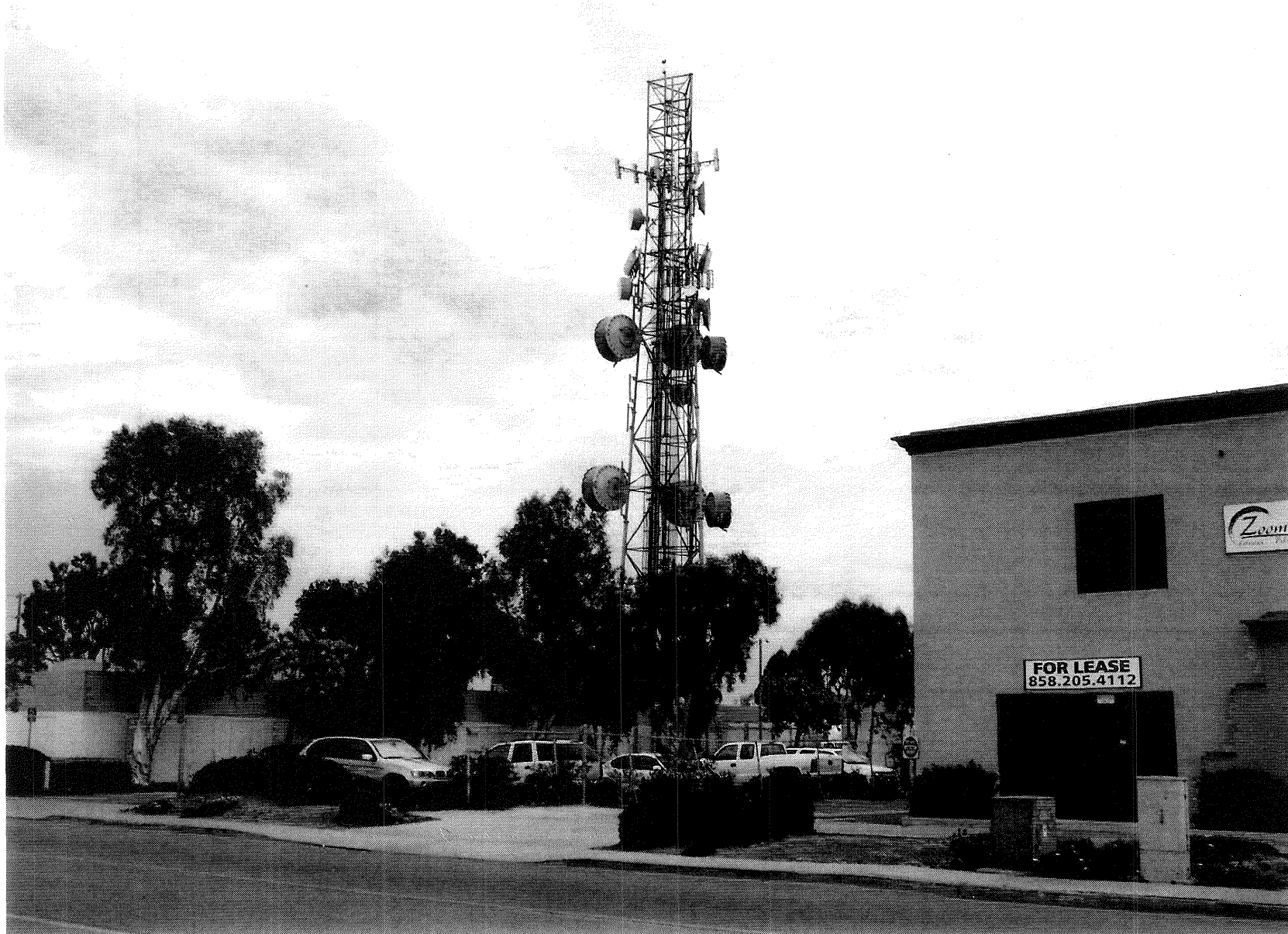
View 2 (Before): View showing existing conditions along the southern boundary of the project site. Verizon Wireless proposes to plant four (4) 36-inch box eucalyptus trees along the southern boundary to match existing landscaping trees for screening.
