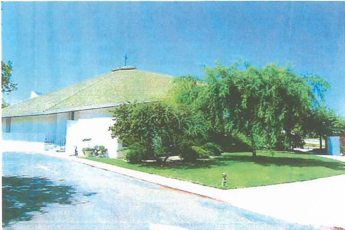
PROPOSED VERIZON EQUIPMENT LOCATION (SPRINT BEHIND NOT VISIBLE)
