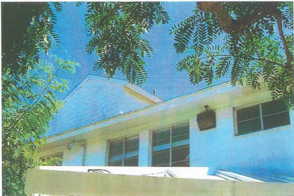
EXISTING SRPINT FACILITY ON SITE
