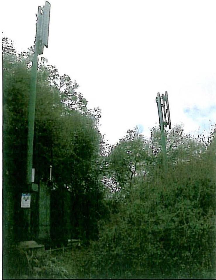
VIEW OF EXISTING ANTENNA MASTS
