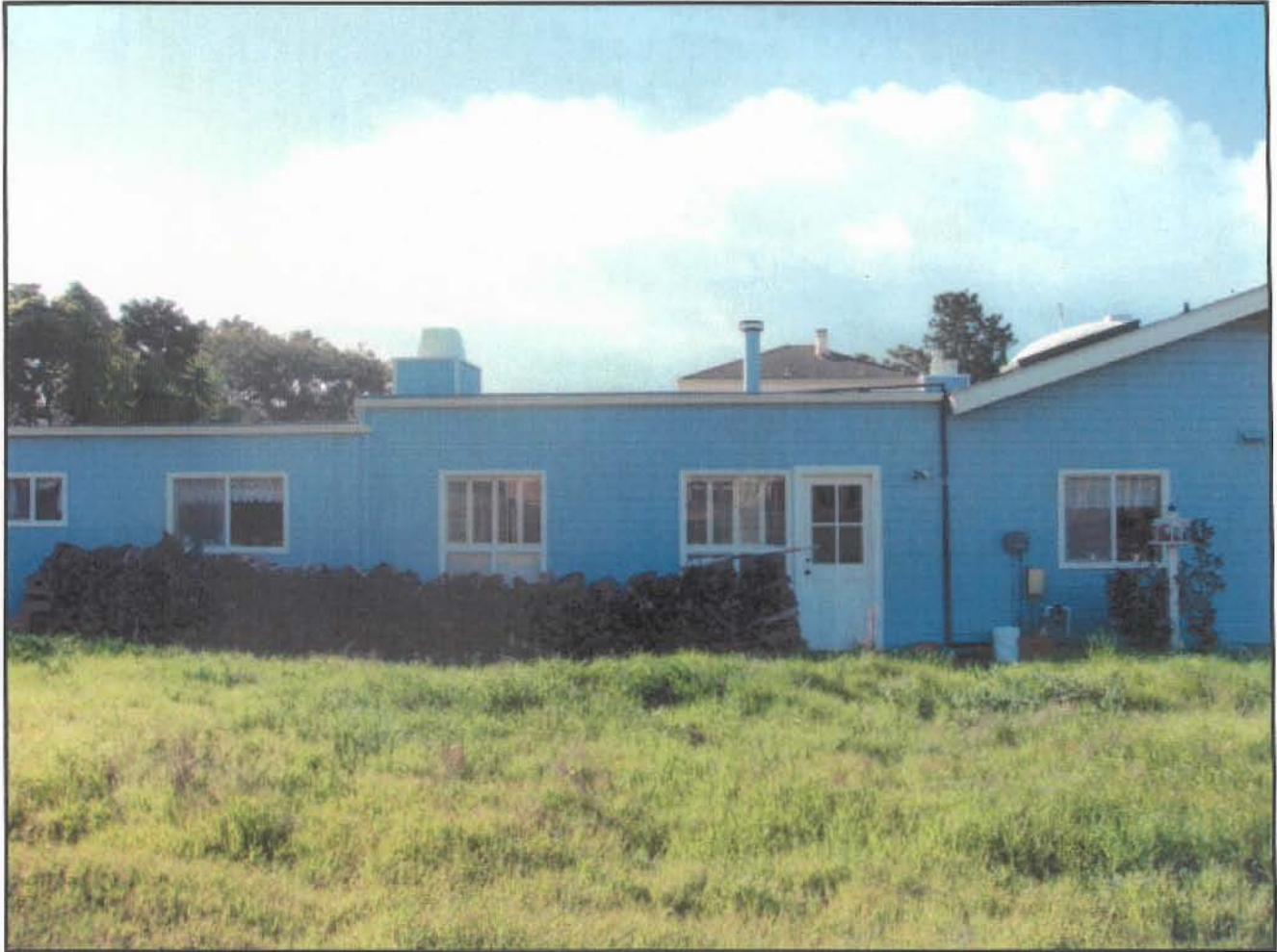
PHOTO #3 -13741 Pine Needles Dr. Deed restricted home to the south. Note roof in background of two story home on the other side.
