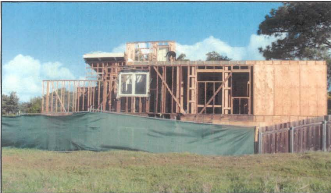
PHOTO #2 - Two story remodel under construction on adjacent property to the north
