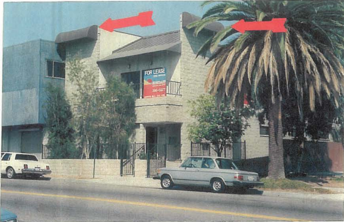
View of building prior to installation of previous wireless facility.
