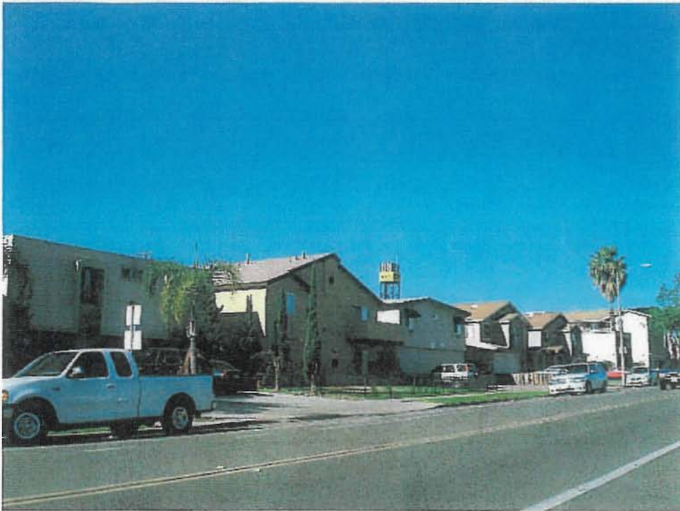
Looking Northwest toward the project
