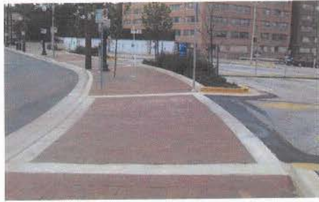
Enhanced Paving at Crosswalk
