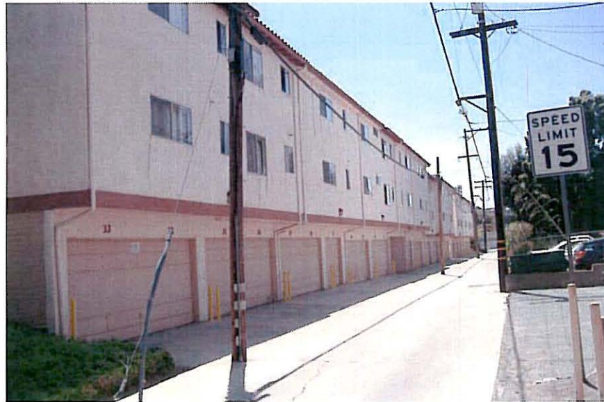
Rear view of units from alley.
