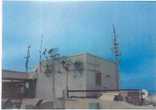
Existing Telecommunications (not Sprint-owned)
