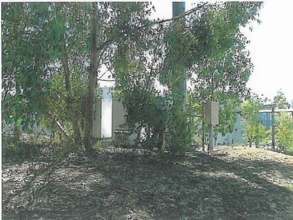
2. Looking at existing equipment and base of pole
