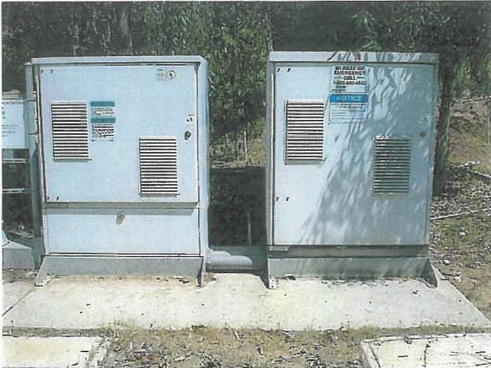
1. Looking at existing equipment cabinets
