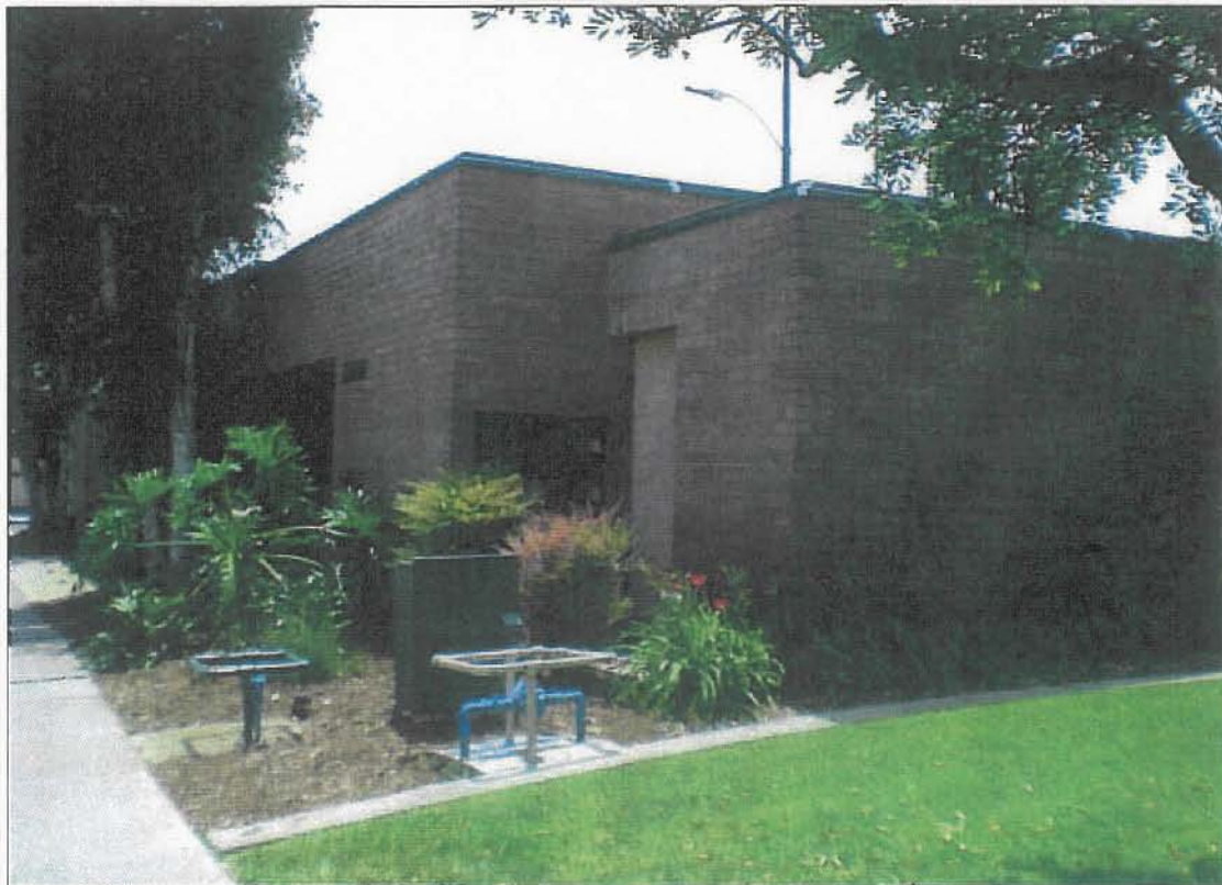
Existing Community Center Building
