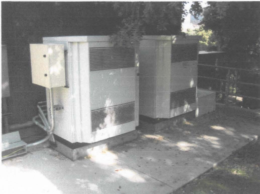
8. View of equipment cabinets.
