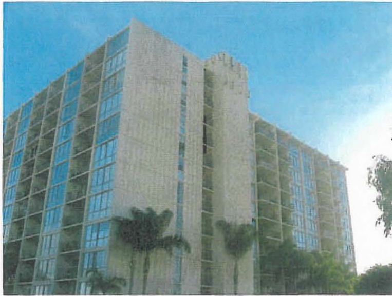
7. Looking at the East elevation of the building
