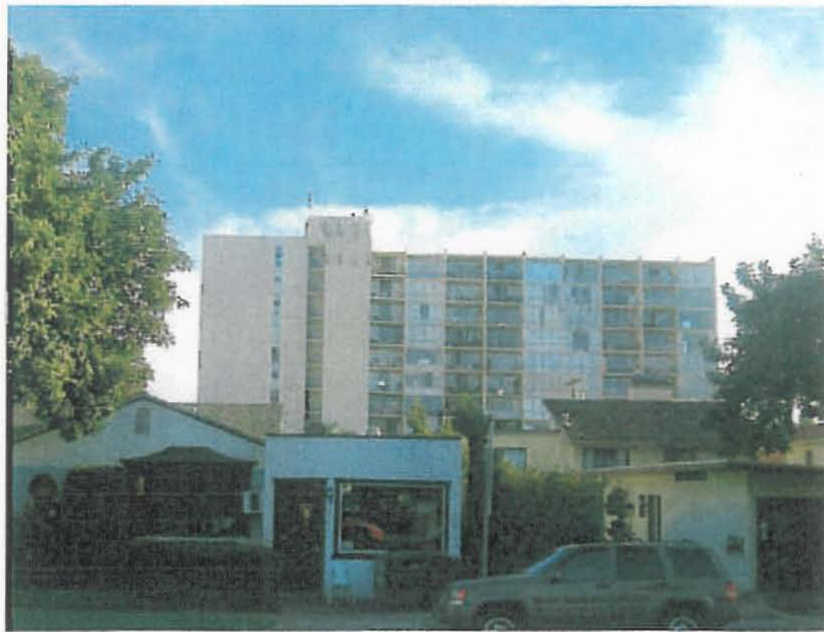
5. Looking at the North elevation of the building
