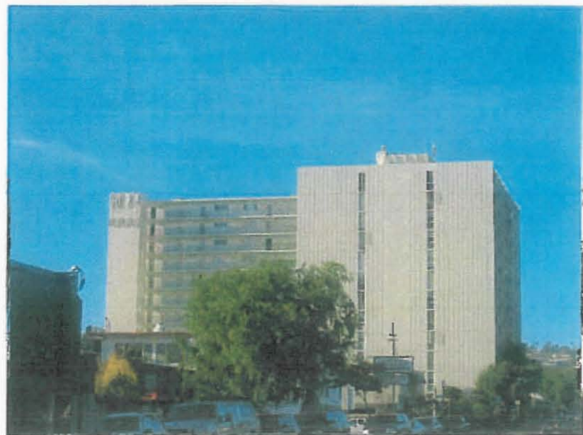
6. Looking at the South elevation of the building
