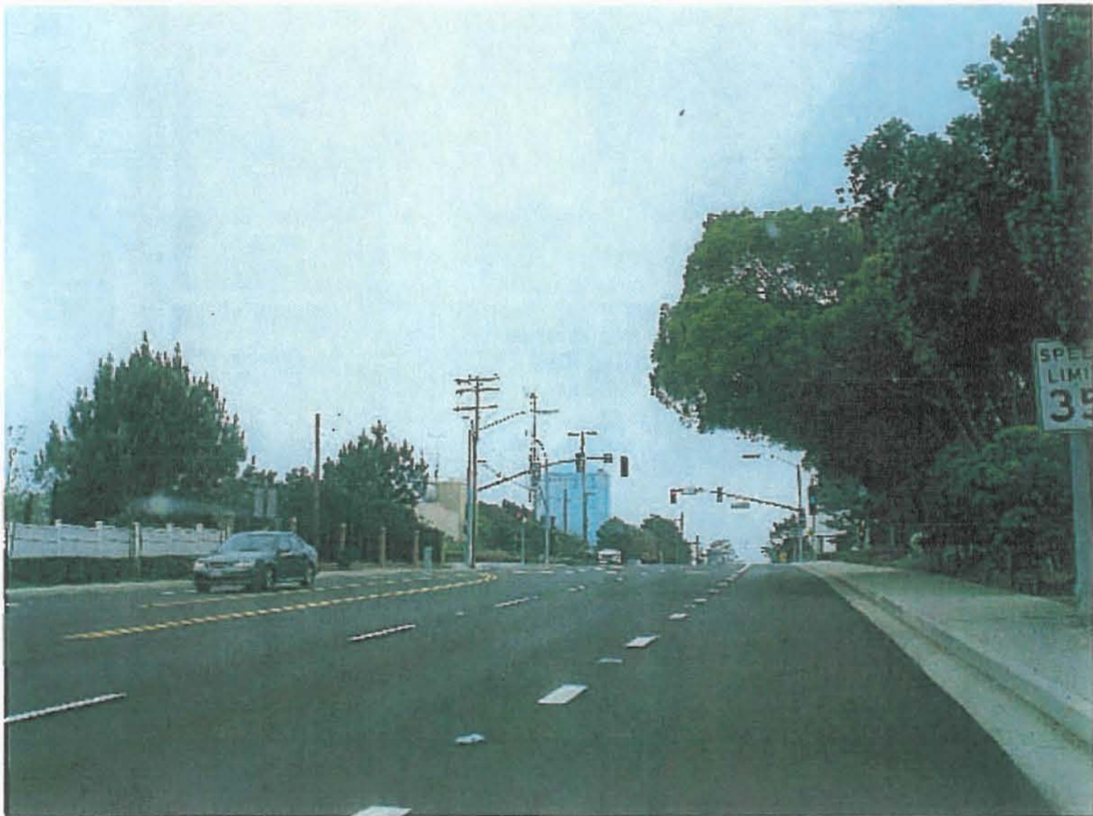
Looking south toward site
