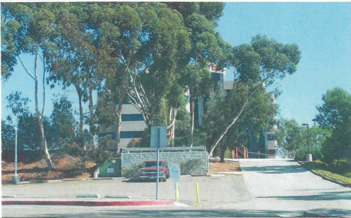
West elevation of building viewed from Annrae St. – AT&T installation screened by landscaping
