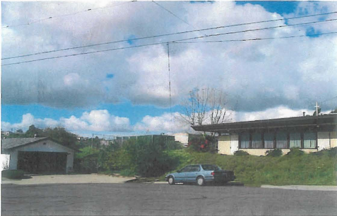
4. East Elevation (not visible)
