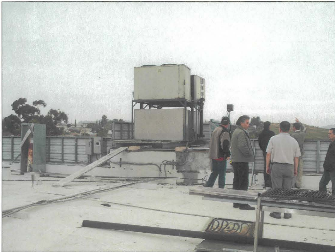
Existing mechanical equipment to be screened as part of VZ Project Proposal.
