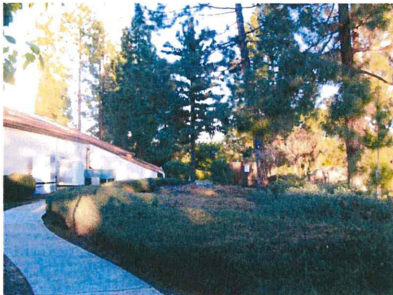
Looking at west elevation
