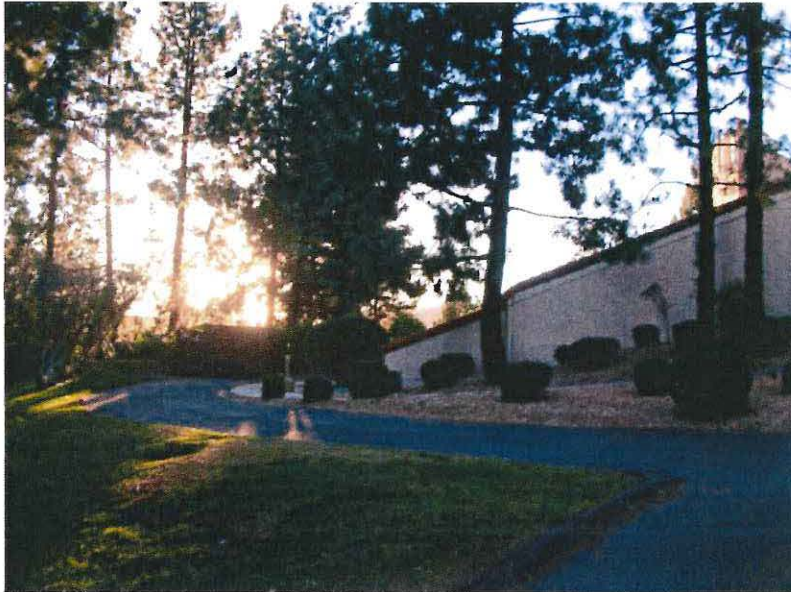
Looking at east elevation
