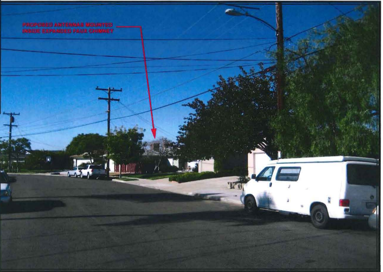
SITE AFTER INSTALLATION
