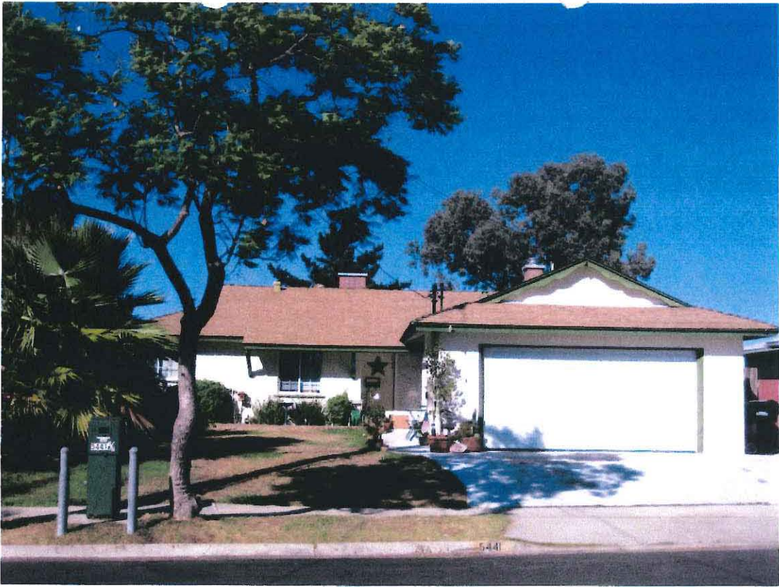
LOOKING NORTHEAST AT SUBJECT PROPERTY
