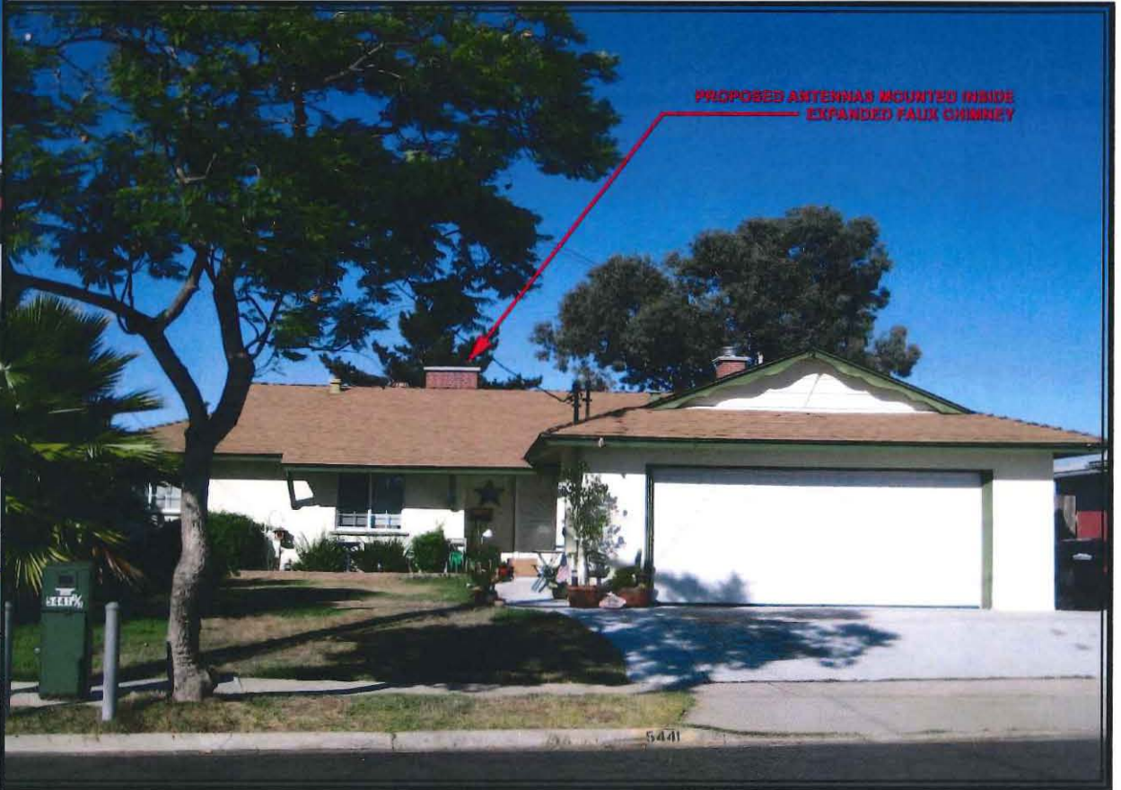
SITE AFTER INSTALLATION
