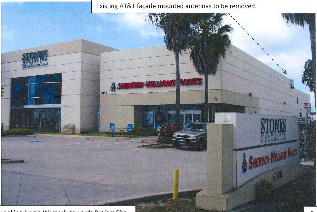
Looking North Westerly towards Project Site
