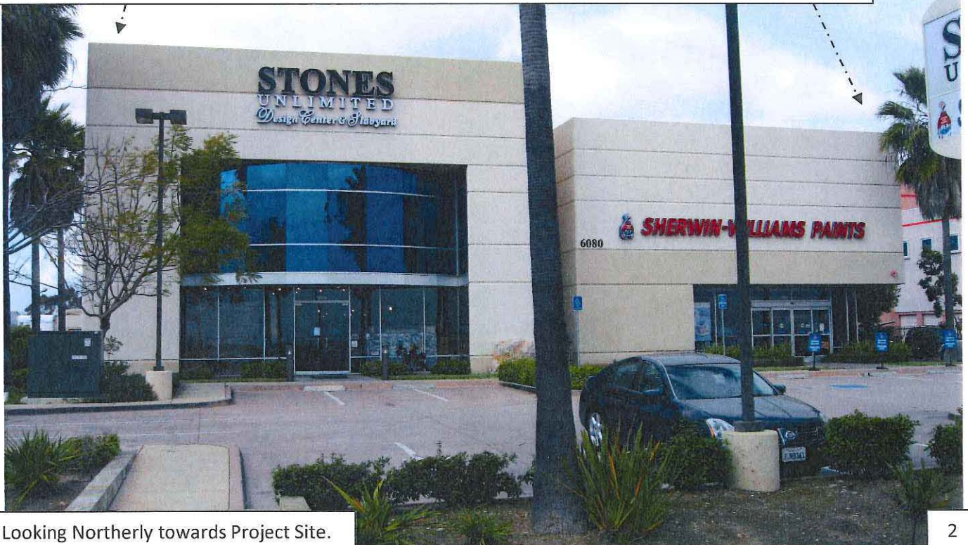
Existing AT&T antennas on rooftop in rear North West corner mounted behind RF screening and façade mounted on the East side of the building (not visible in this view).
