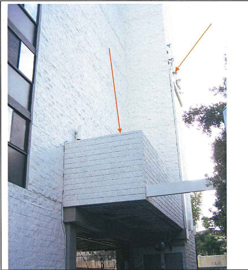
AT&T equipment enclosure and north antenna sector
