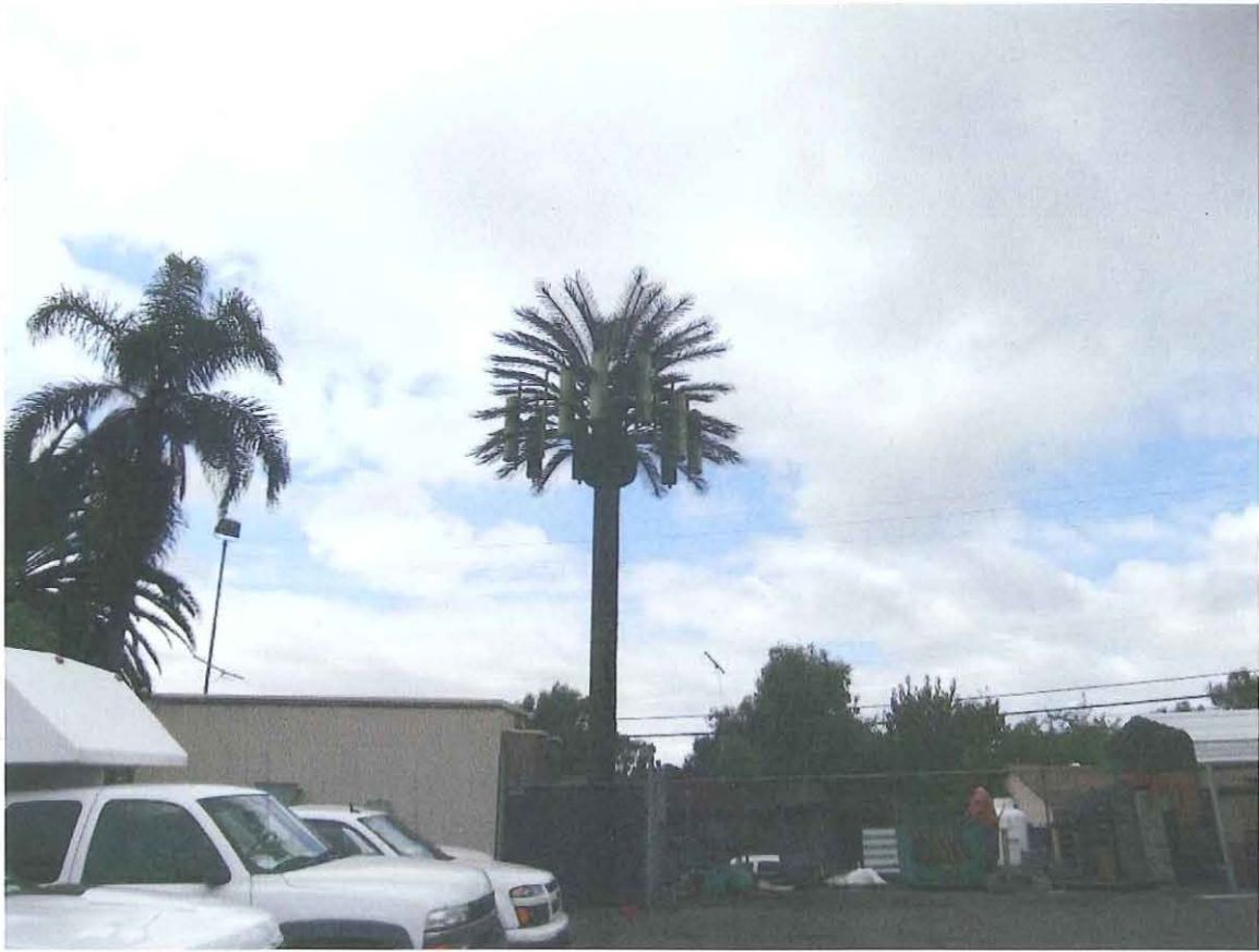
Looking West towards existing monopalm and equipment shelter.
