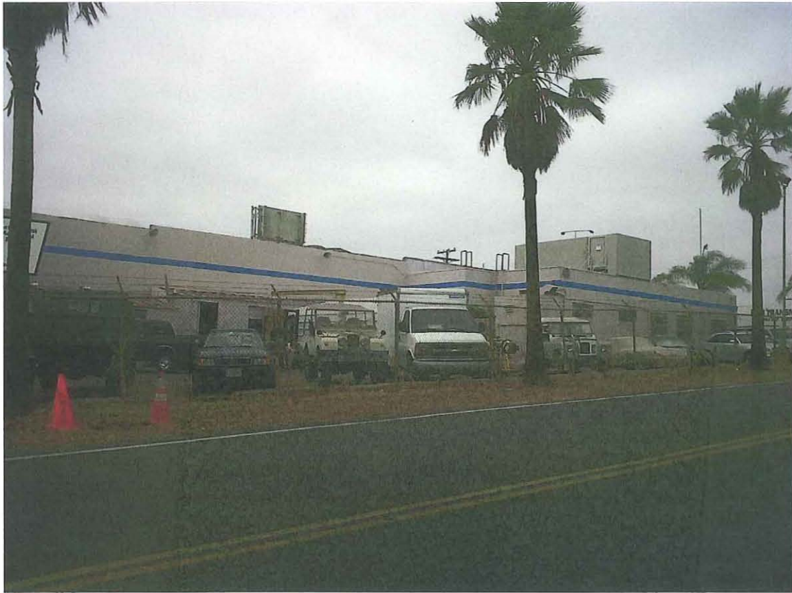
7. Looking East at existing building with rooftop WCF.
