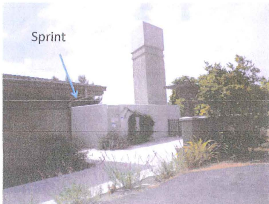
Equipment location inside CMU wall and slatted gates
