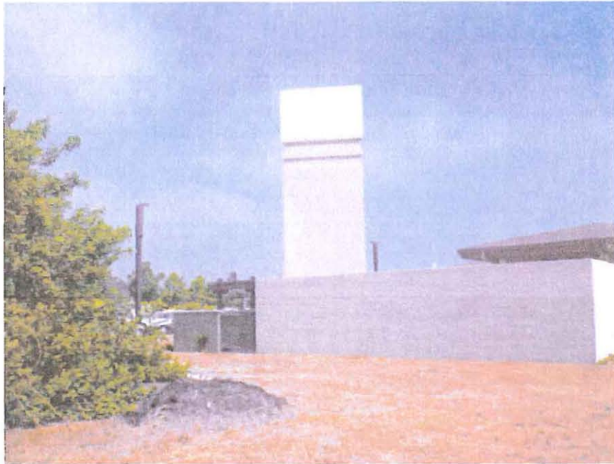
View of south sector looking north
