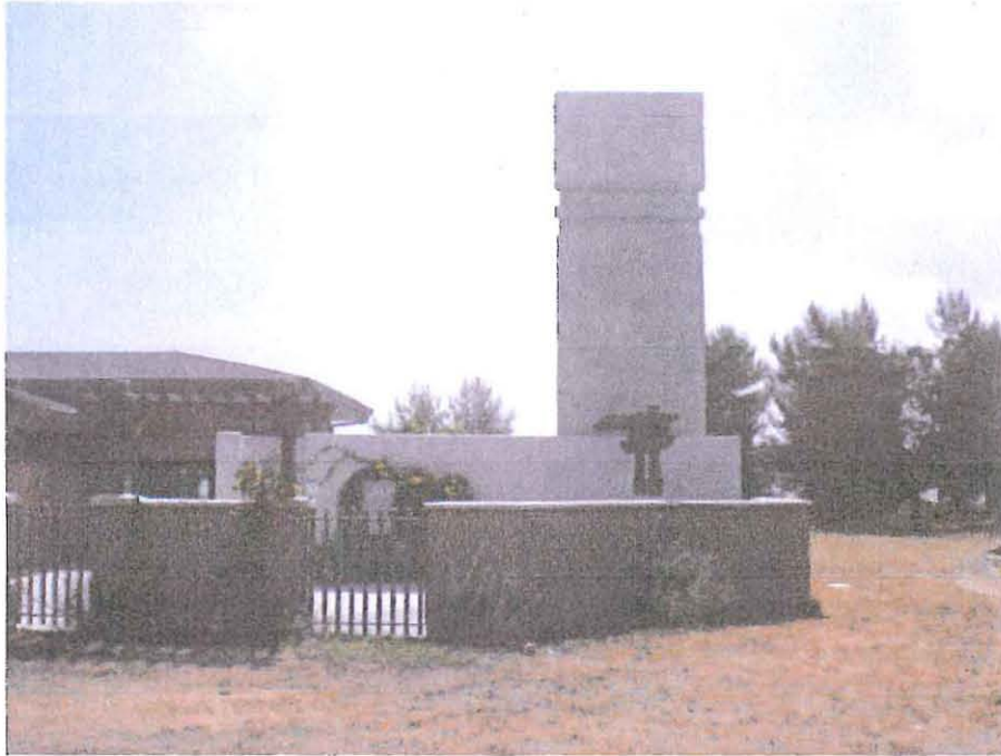
View of site and tower from the west
