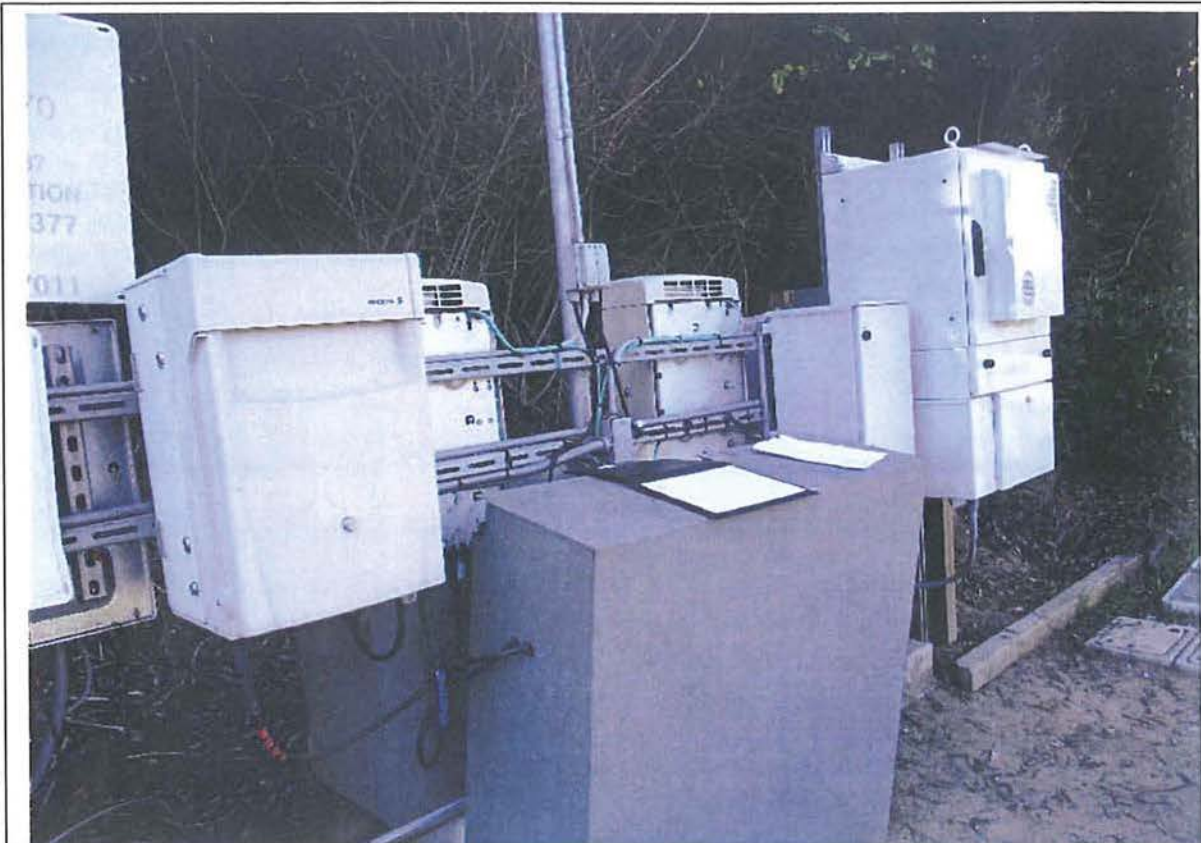
AT&T base station area
