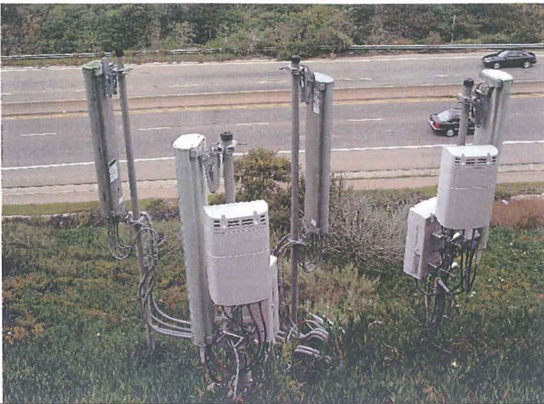
AT&T post-mounted antennas
