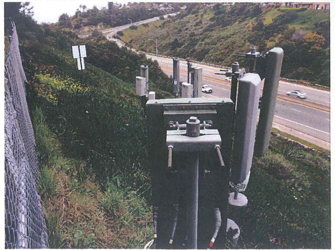
AT&T antennas in background and Verizon antennas in foreground
