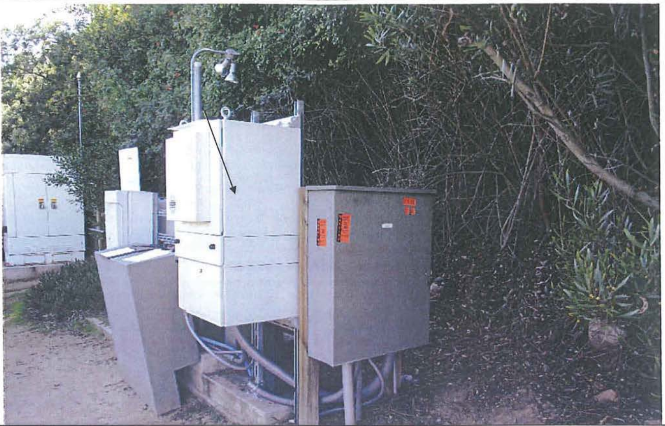
AT&T base station area
