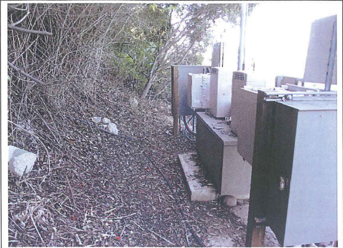
Back side of AT&T base station area
