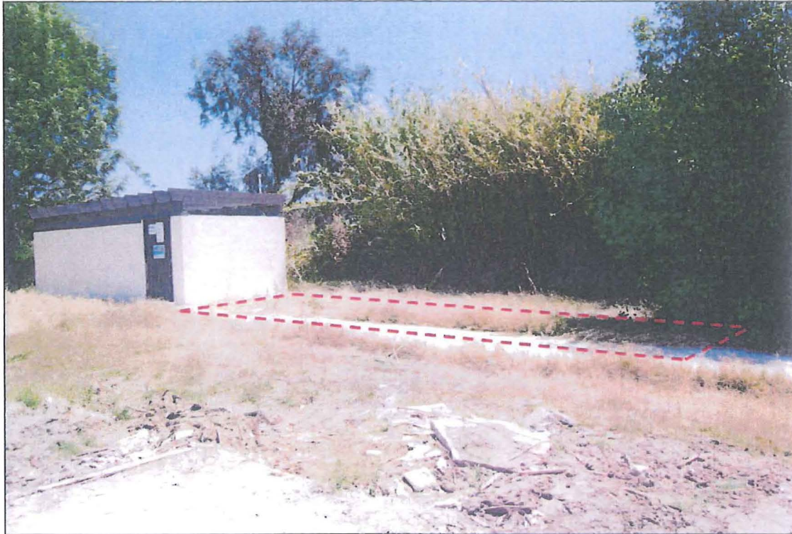
Verizon Tree/Equipment Area
