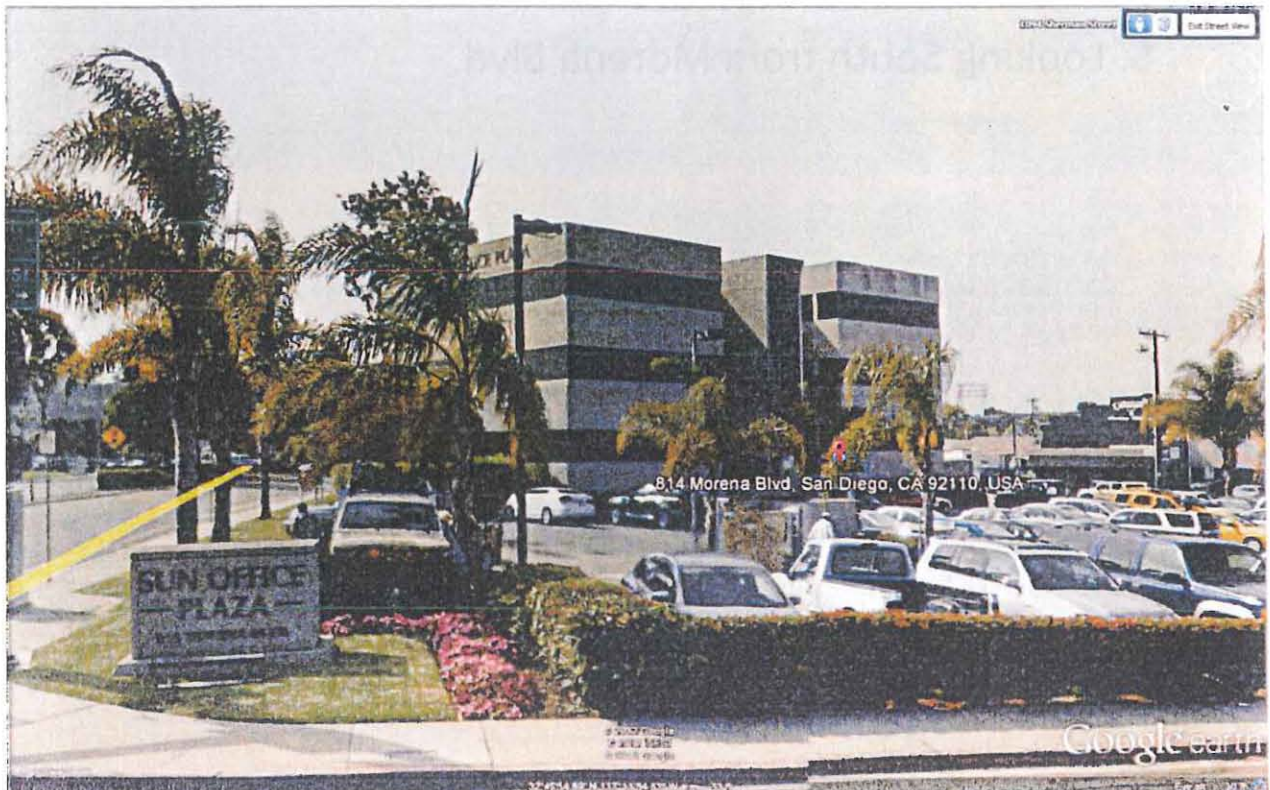
4. Looking South from intersection of Morena Blvd and Sherman St.
