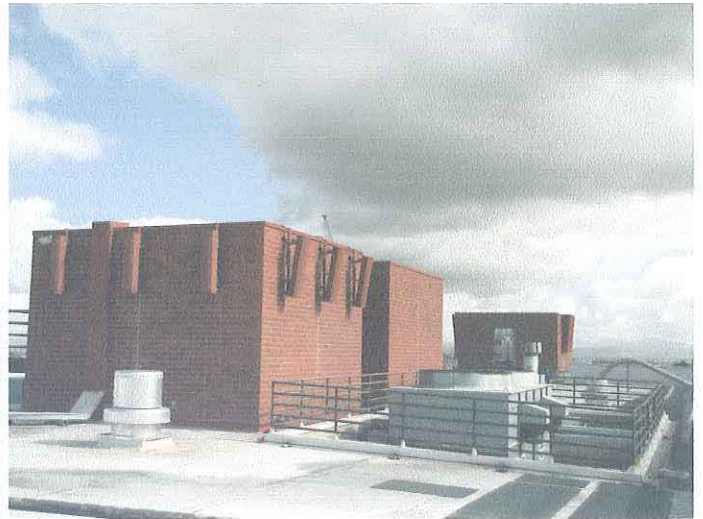
6. East facing view of existing antennas
