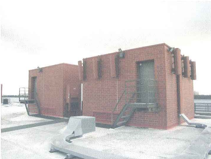
5. South facing view of Sprint PCS antennas
