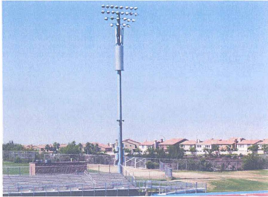
Looking at existing site
