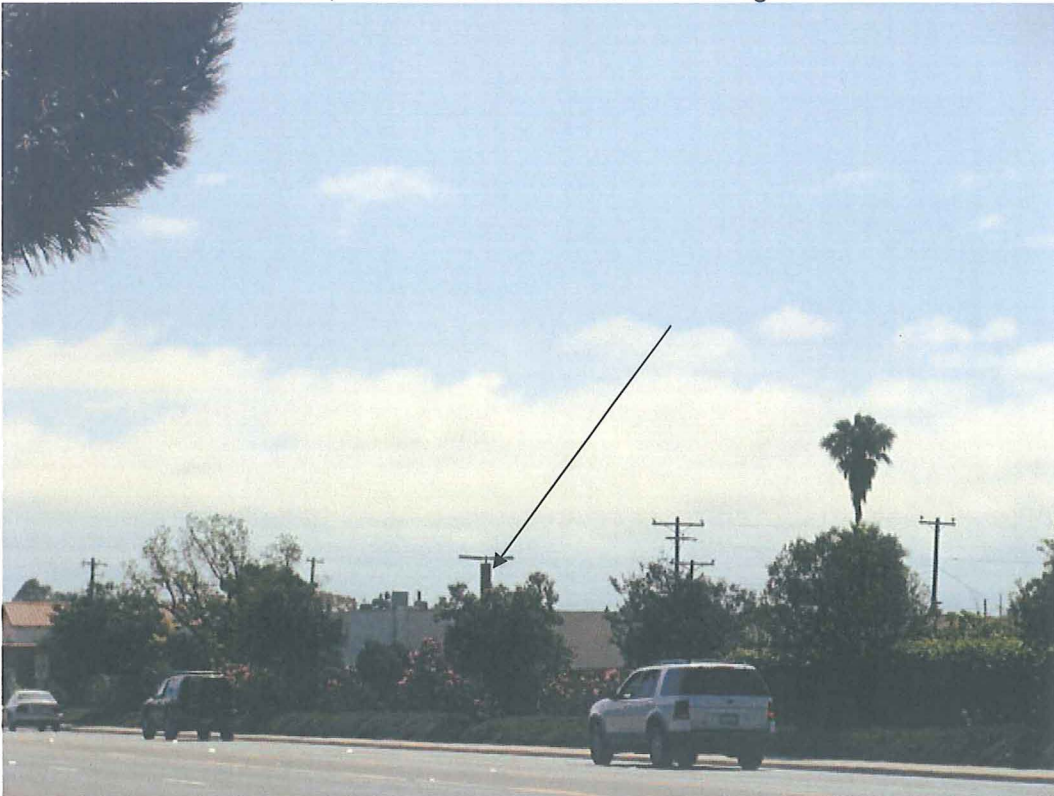
East elevation of antennas from across Linda Vista Road; one sector not visible
