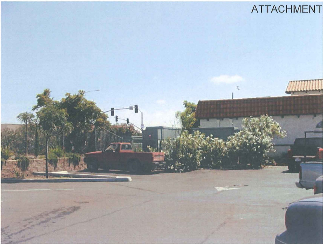
North elevation of equipment
