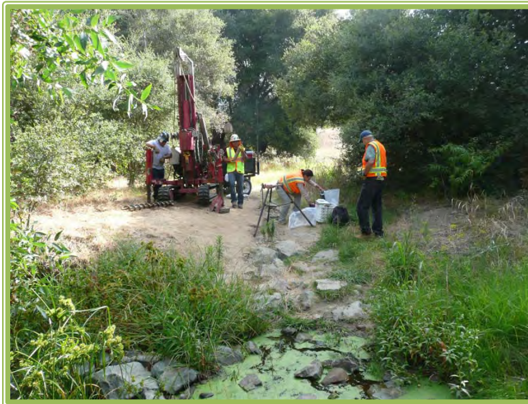
North Tecolote Canyon – Geotechnical Sampling Near Crossing
