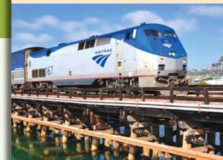
The San Dieguito Double Track rail project will provide direct access to the Del Mar Fairgrounds for COASTER and Amtrak passengers.
