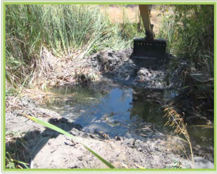
San Diego Mission Road MH 111 Emergency Raising & Cleaning
