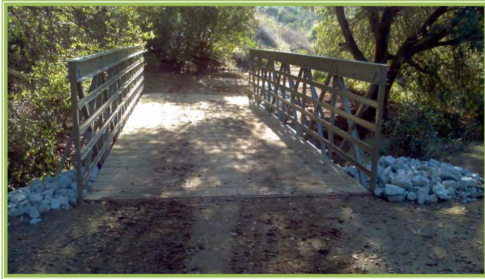
Mt. Elbrus Canyon- New Access Bridge
