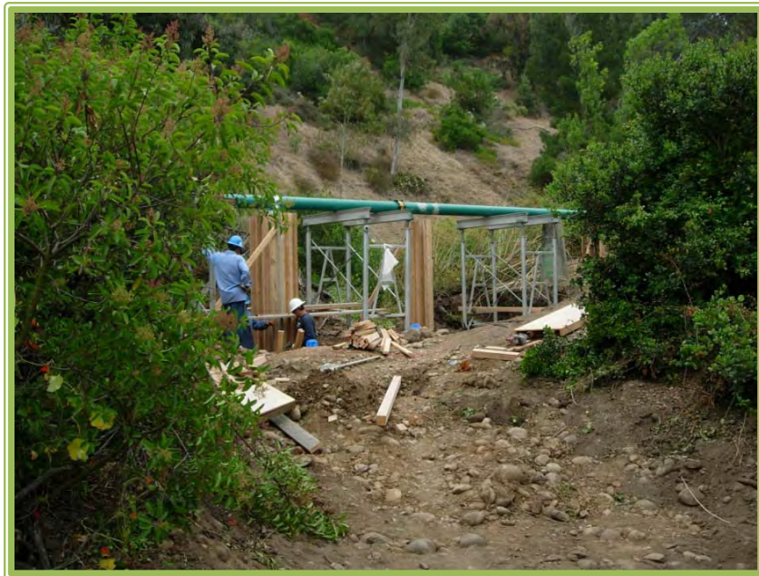
Hotel Circle South Emergency Pipe Pillar Replacement
