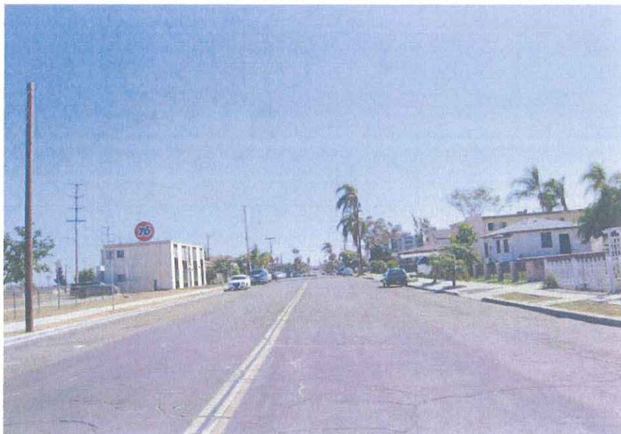
Looking south from site
