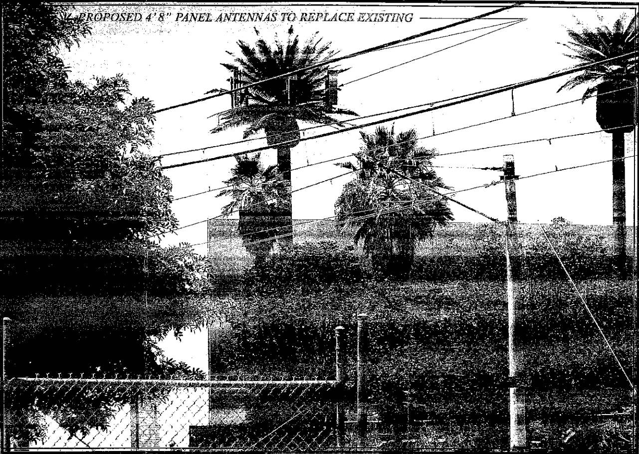
SITE AFTER INSTALLATION
