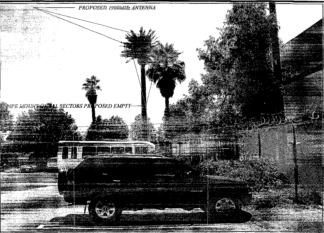
SITE AFTER INSTALLATION
