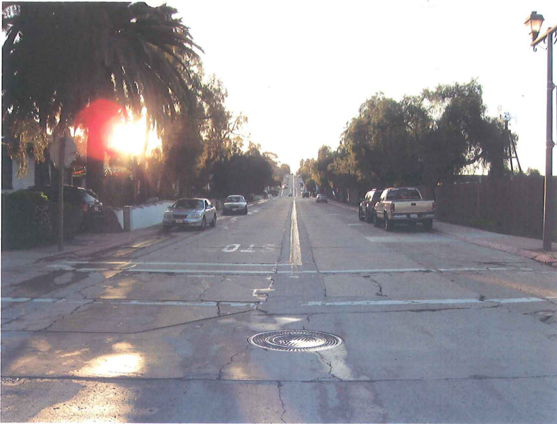
Juan St @ Mason St – Looking southeast towards Twiggs St
