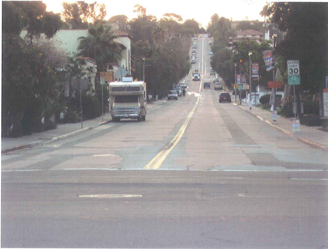
Juan St @ Taylor St – Looking southeast towards Wallace St
