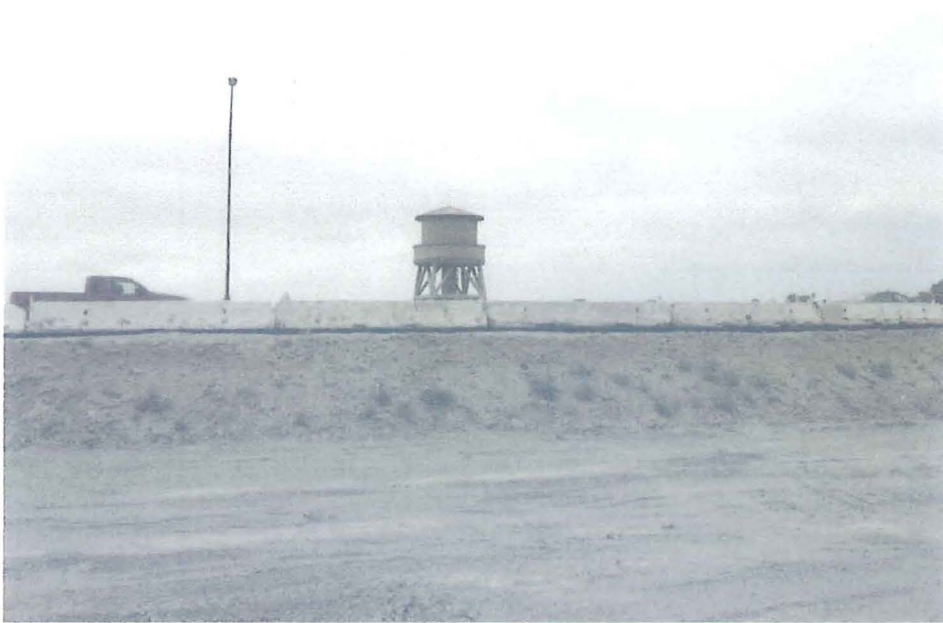
(1) View of the subject property looking north.
