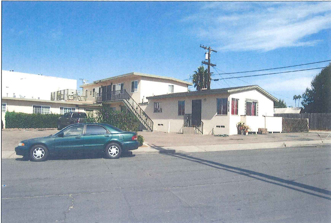
View Looking North
