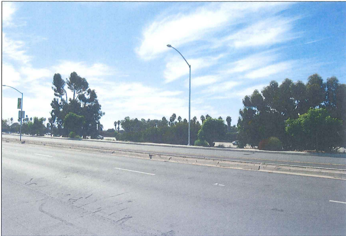
View Looking Southwest
