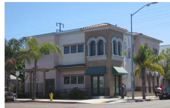
A wide variety of industrial and commercial uses occupy nearly 270 acres of land in Southeastern San Diego.
