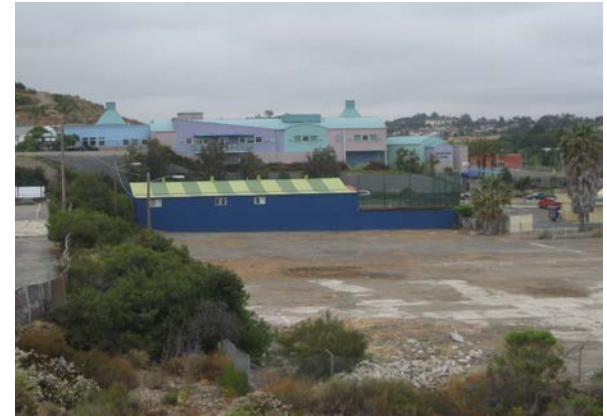
View of Focused Improvement Area 2 from Guymon Street
