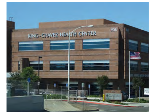
The 3-story, 25,000-square foot King-Chavez Health Center opened in September 2012.
