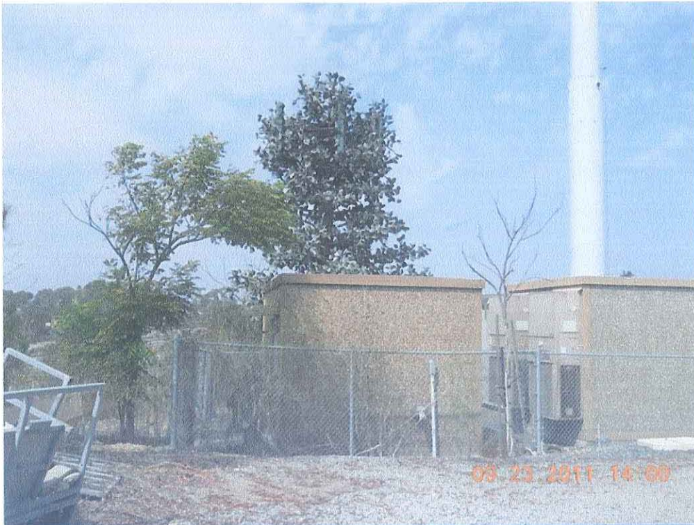
1. View from the south
