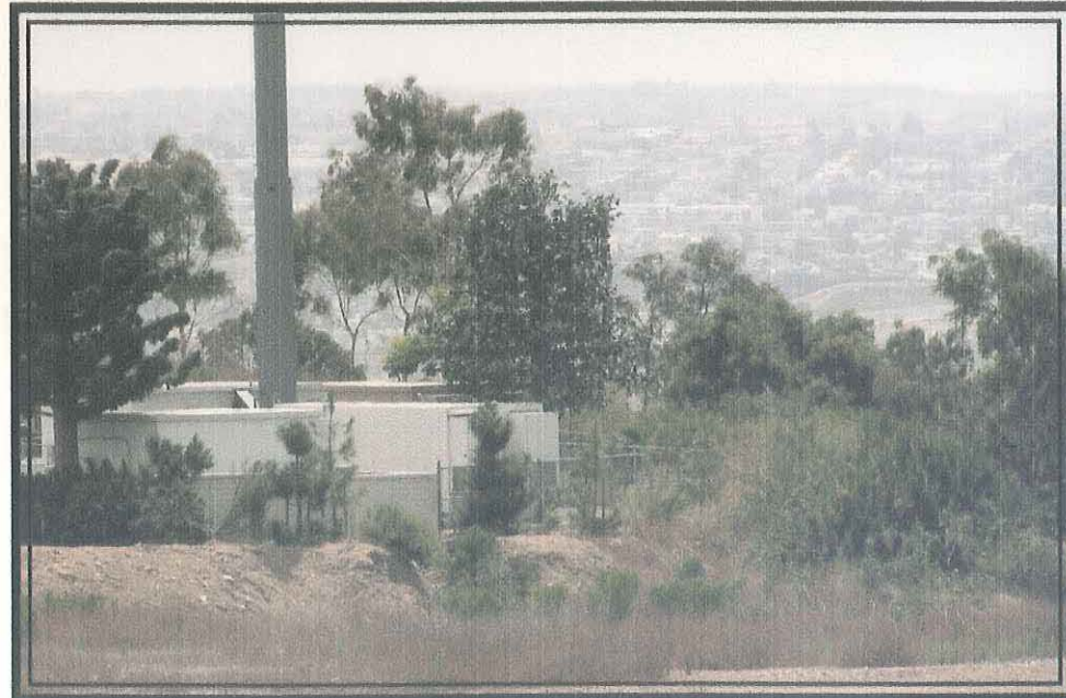
SITE PRIOR TO INSTALLATION
