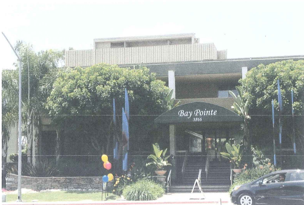
AT&T BAY POINTE PHOTO SURVEY
