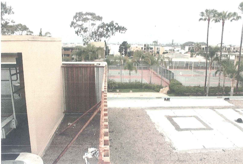
AT&T BAY POINTE PHOTO SURVEY
