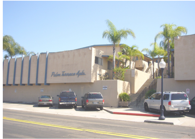
Existing Apartment Building (before)
