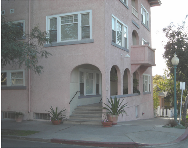
A multi-family apartment building in the community that addresses the street corner with steps and an arcade at the building entrance
