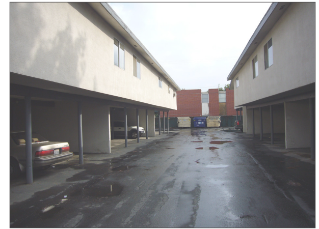
Unimproved alley (before)
