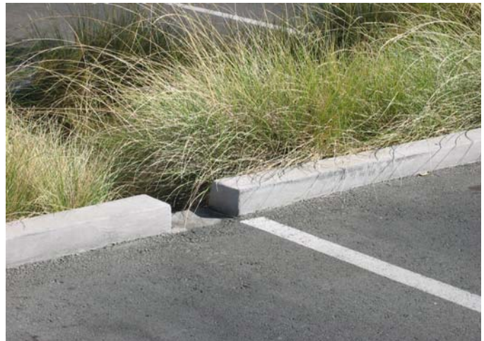
The use of sustainable site design elements aid in reducing stormwater runoff.
