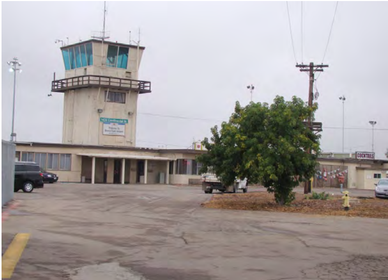
Photo No. 1 Area 1 - Administration and control tower building at 1424 Continental Street in the central portion of the Brown Field operations area (Map ID 2)
