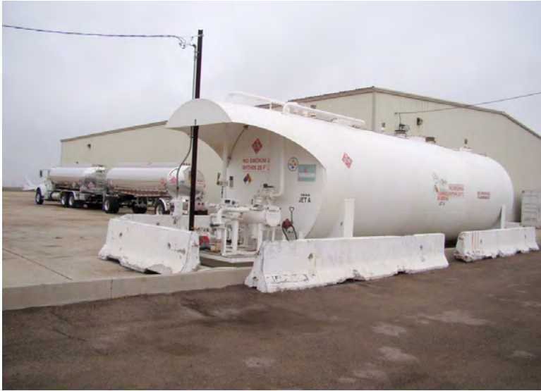
Photo No. 5 Area 1- ASTs containing jet fuel south of the hangars in the Brown Field operations area (Map ID 2)
