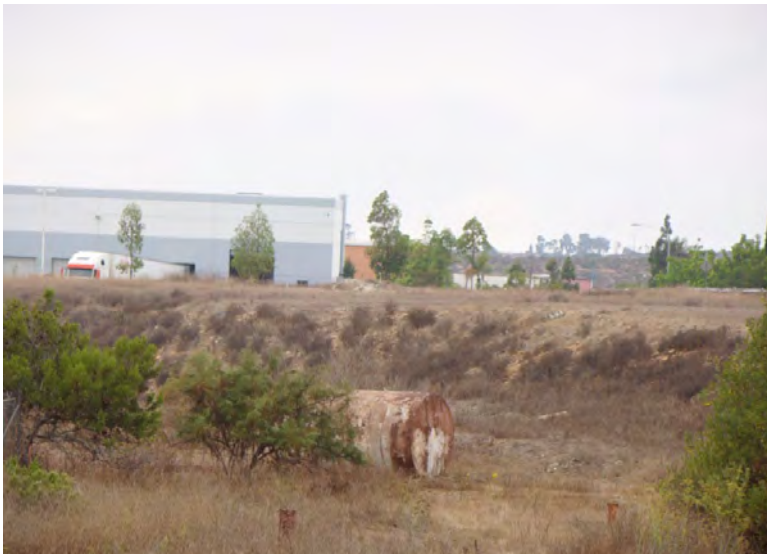
Photo No. 23 Area 3 – Abandoned aboveground storage tank observed in the western portion of the Sesi Property (Map ID 17)
