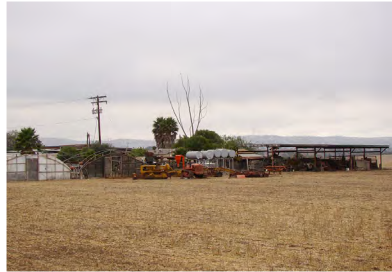
Photo No. 26 Area 3 – Diesel aboveground storage tanks observed in the northern portion of the Martinez Ranch Compound (Map ID 18)
