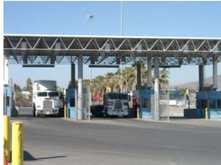
Truck Inspection at Otay Mesa POE
