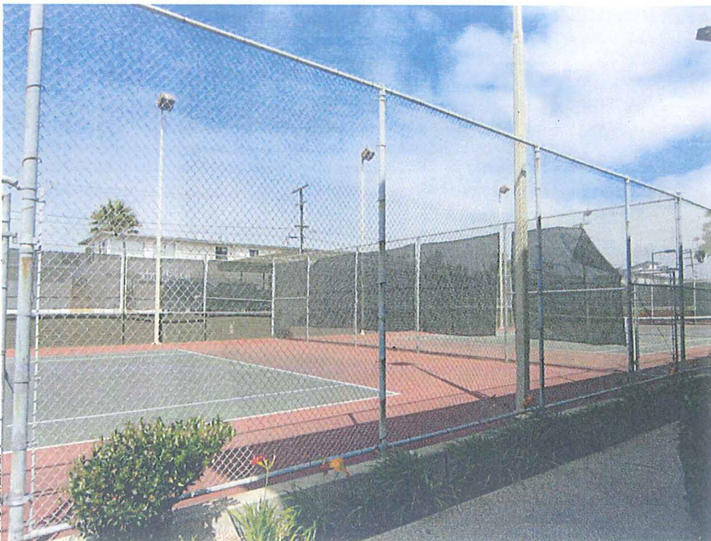
(6) View from the subject property looking west.
