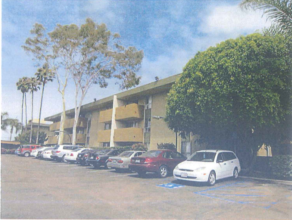
(1) View of the subject property looking north.
