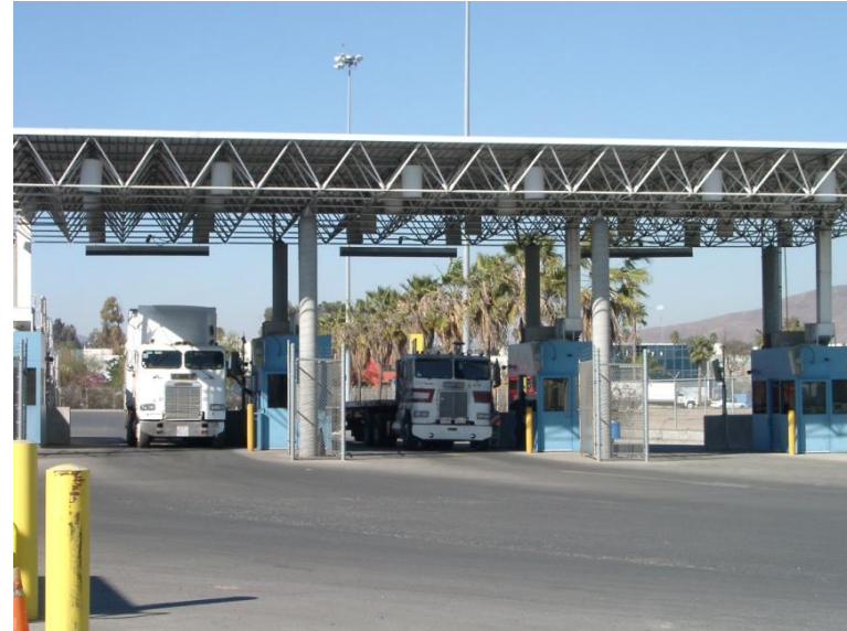
Truck Inspection at Otay Mesa POE
