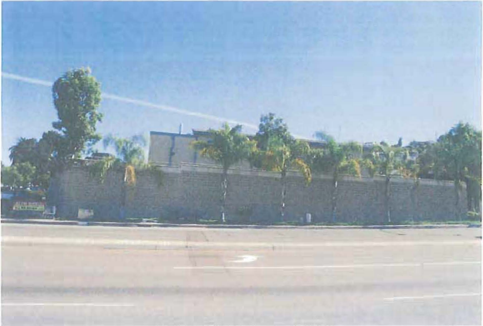
Looking at west elevation
