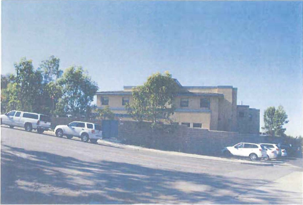
Looking at east elevation
